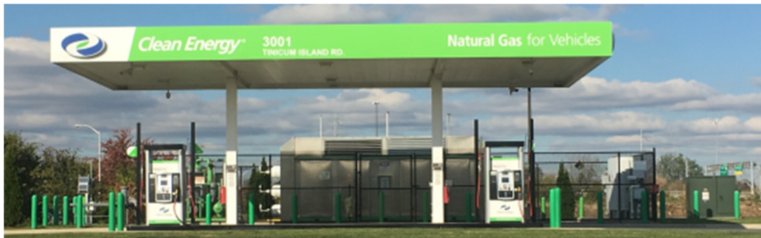
Figure 3 – “Wally Park” CNG Fueling Station at Philadelphia Airport
