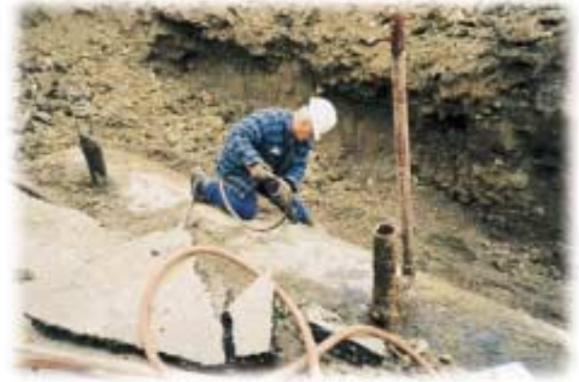
A cleanup team member prepares a storage tank for removal.
