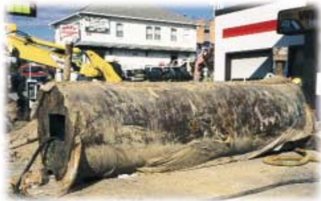
An example of the type of storage tank removed from properties across Pennsylvania.
