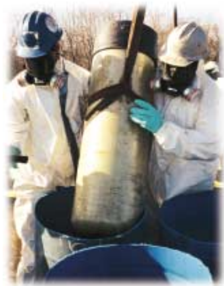
Remediation workers overpack a drum for cleanup purposes.
