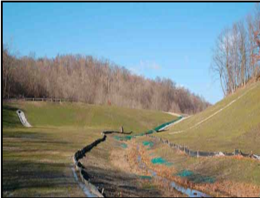
Figure 7 – Upstream segment of re-constructed stream channel (upper left), middle segment of channel showing willow plantings in riparian area (upper right), lower segment of channel showing re-contoured highwalls (lower left), and the Fishing Run stream channel below the site.
