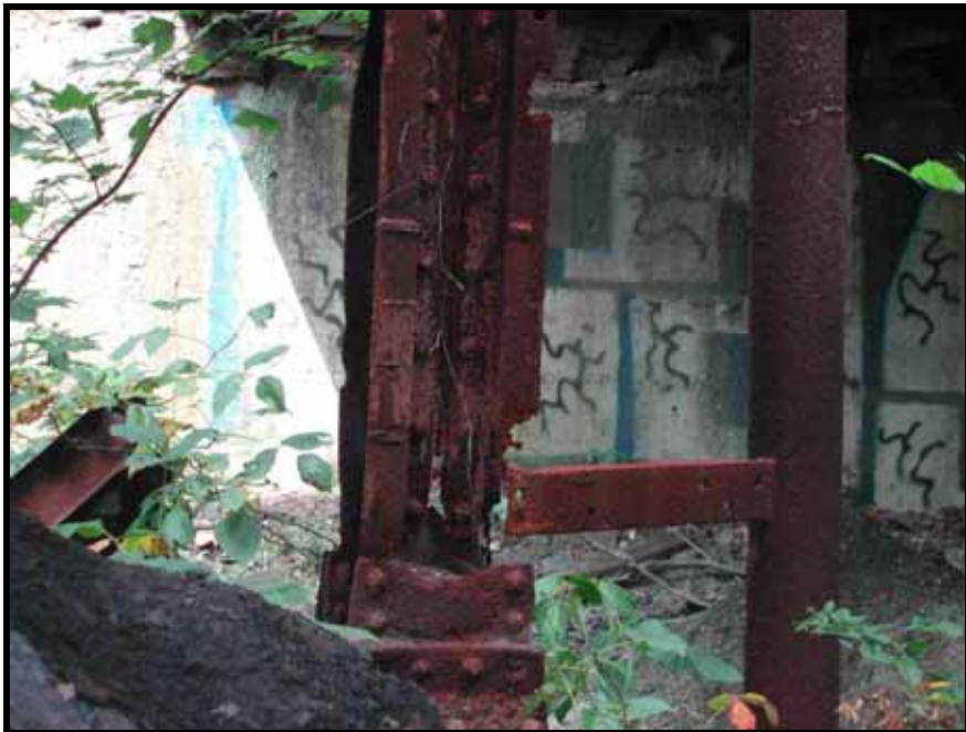
Figure 4 – Hazardous tippel and bin structure (upper left), dangerous highwall (upper right), deteriorated steel column and graffiti on tippel structure (lower left), and entire flow of Fishing Run entering the open mine entry.
