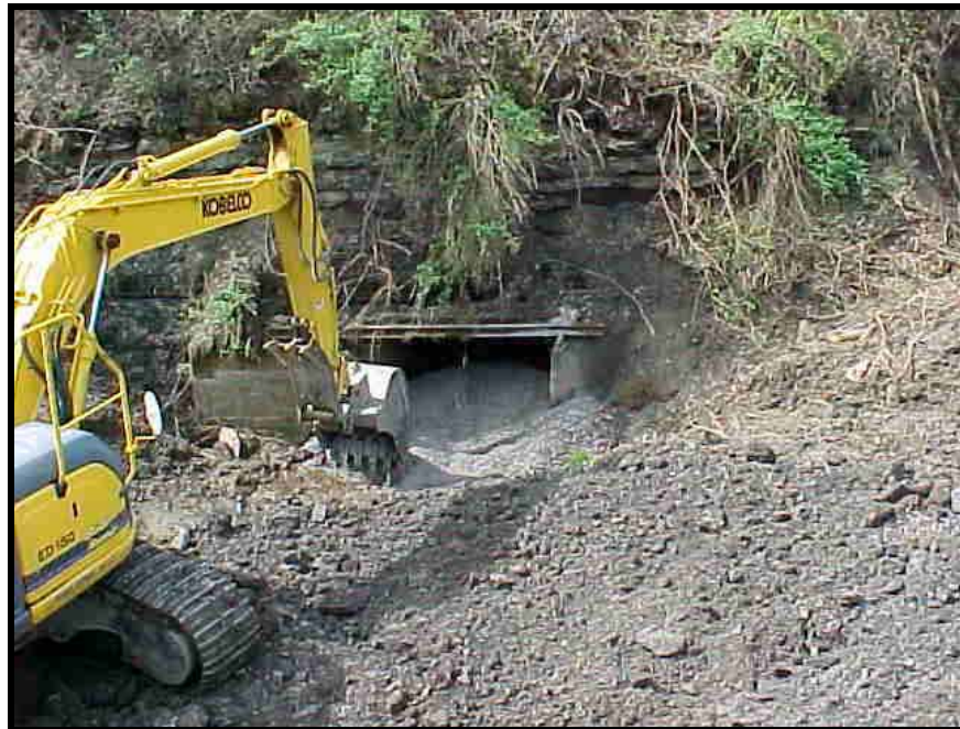
Figure 5 – Initiation of project construction (upper left), construction of the first segment of the new Fishing Run stream channel (upper right), sealing of open mine entry (lower left), and backfilling of dangerous highwall with borrow material (lower right).
