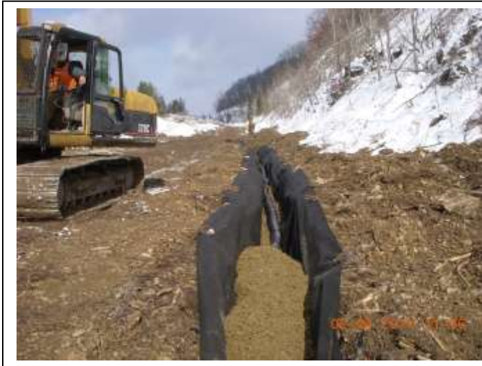
Installation of the subsurface drain.
