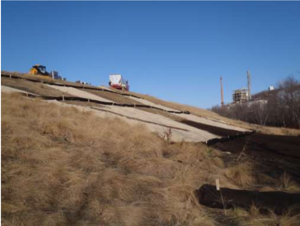
Post-reclamation – installing compost filter socks & compost blankets & seeding
