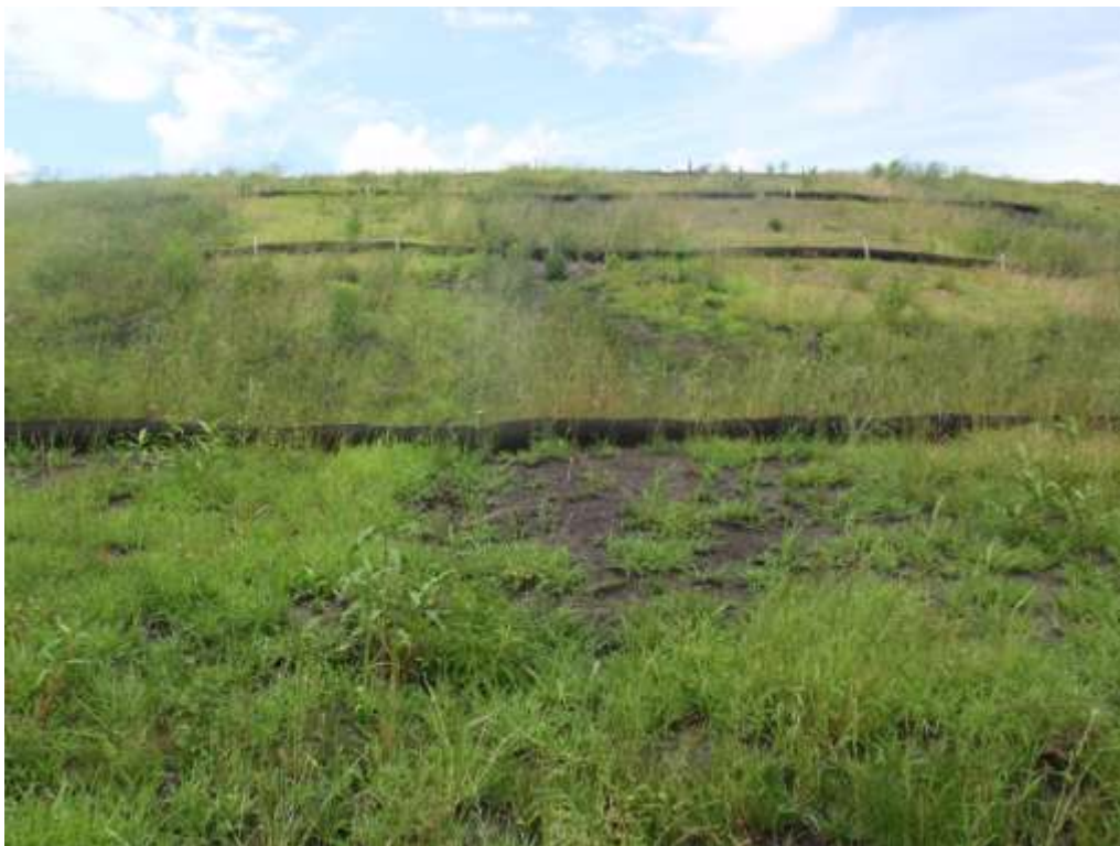
Post-installation of compost filter socks & compost blankets & seeding
