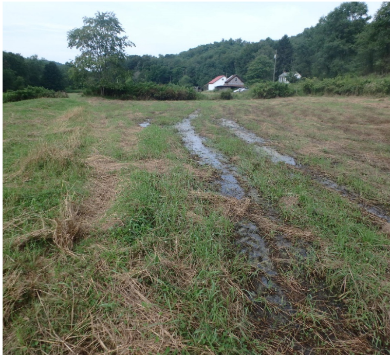
Figure 6-6. Ponding in low area over Cumberland Mine (Photograph taken from PADEP file).
