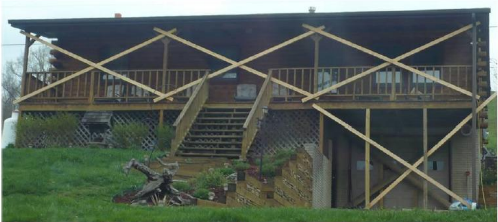
Figure V-14 - Photograph of bracing (photograph courtesy of N. Iannacchione).
