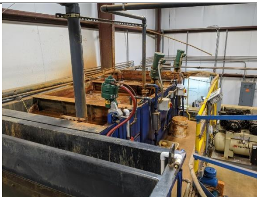
Aeration / Reaction / Flocculation Tanks
