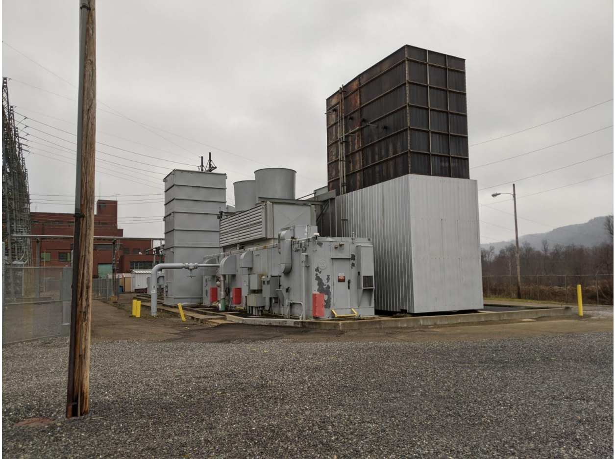
Combustion Turbine (CT) facility owned by Warren Generation LLC. (Photograph taken on 12/4/2019) The CT is a 57-megawatt natural gas- and distillate fuel oil-fired electric generating station, which consists of one operational simple-cycle CT and ancillary equipment and systems. Fuel for the CT is delivered by pipeline (natural gas) and tanker truck (oil).
