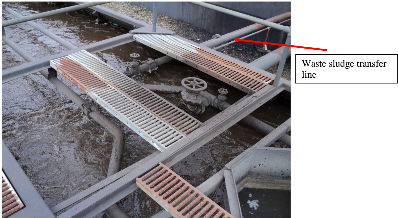
Figure 4: The waste sludge transfer line to move domestic waste sludge to the industrial side aeration tank.
