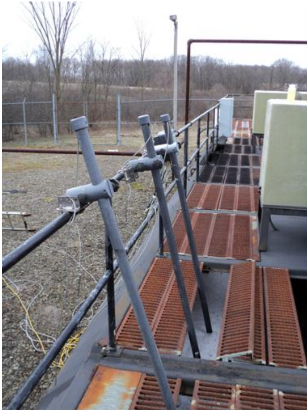
Figure B.1: Photo showing example of online monitoring equipment installed on the industrial train. Much of the grating throughout the facility is heavily rusted similar to that shown in the picture.
