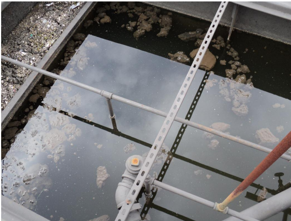
Figure 1: Photo of clarifier for the domestic sewage plant.
