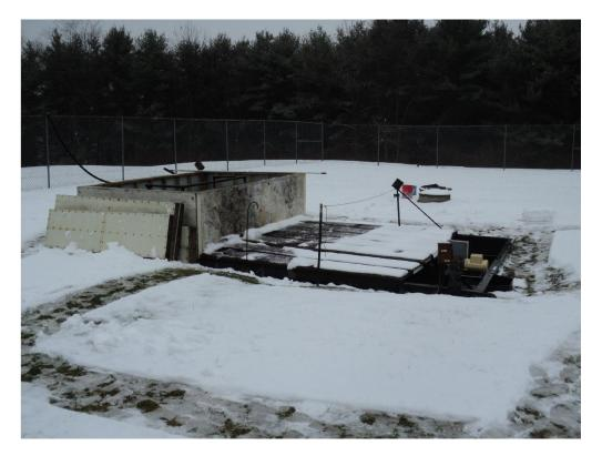
The treatment plant consists of a comminutor, aeration tank, clarifier, chlorine contact tank and sludge holding tank. Sludge solids are removed in liquid form via waste hauler.
