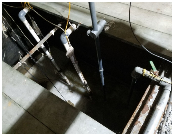
Surge Tank Lift Pumps & UVAS Probe
