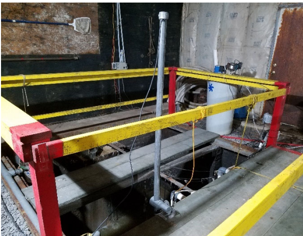
TOC Probe at Surge Tank
