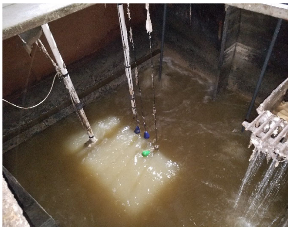
Surge Tank showing corrosion
