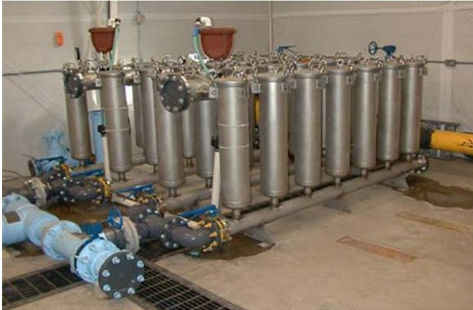
Figure 3.1 An Example of a Multiple Train Filter System Installed at Paonia, CO<sup>1</sup>
