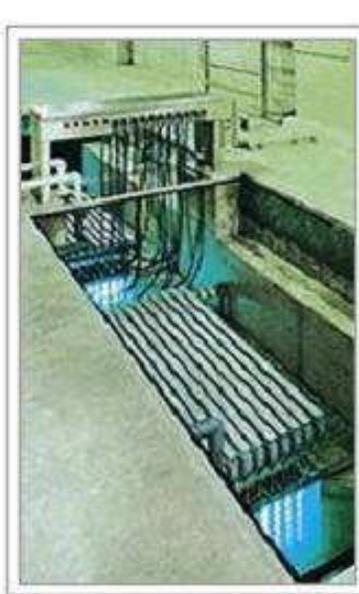
Figure 2.1 An Open Channel Reactor<sup>1</sup>
