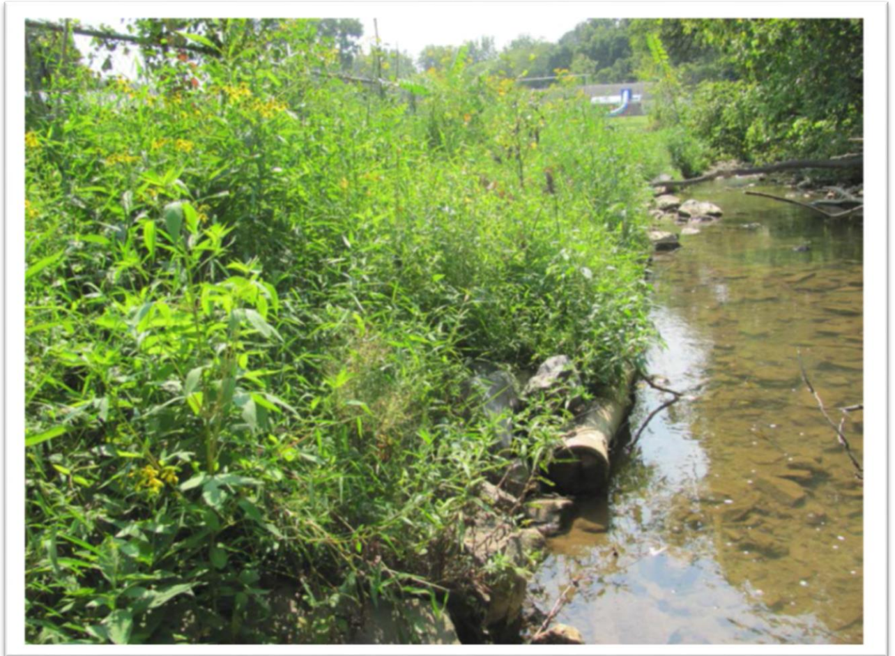
A photo of a mudsill constructed for fish habitat and other benefits as part of project 1315.
