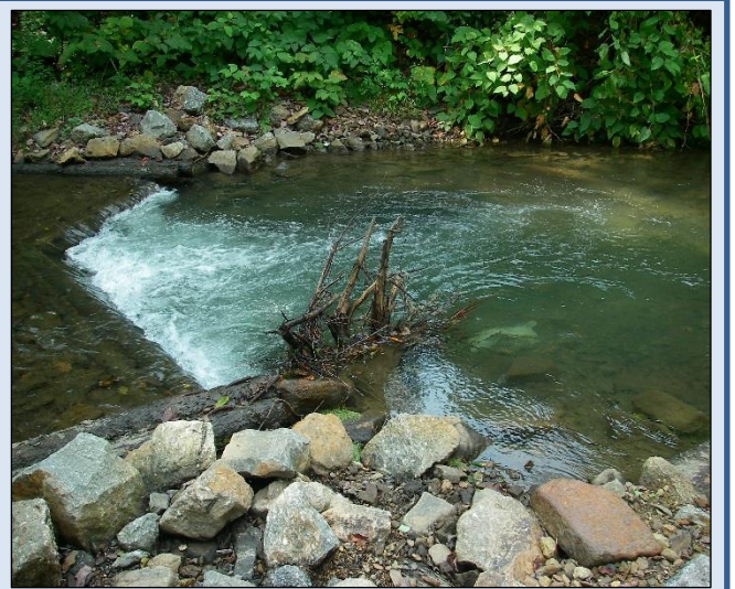
A Log Framed Stone Deflector (left) and a Plunge Pool (right) constructed as part of this volunteer-led habitat improvement project. The installation of these BMPs would have been futile had it not been for the dedicated NPS reduction efforts focused on this watershed years prior.
