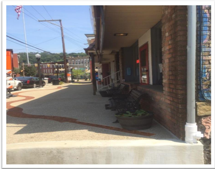
A photo of a sidewalk in Etna Borough with an artistic and decorative stormwater management/infiltration BMP.
