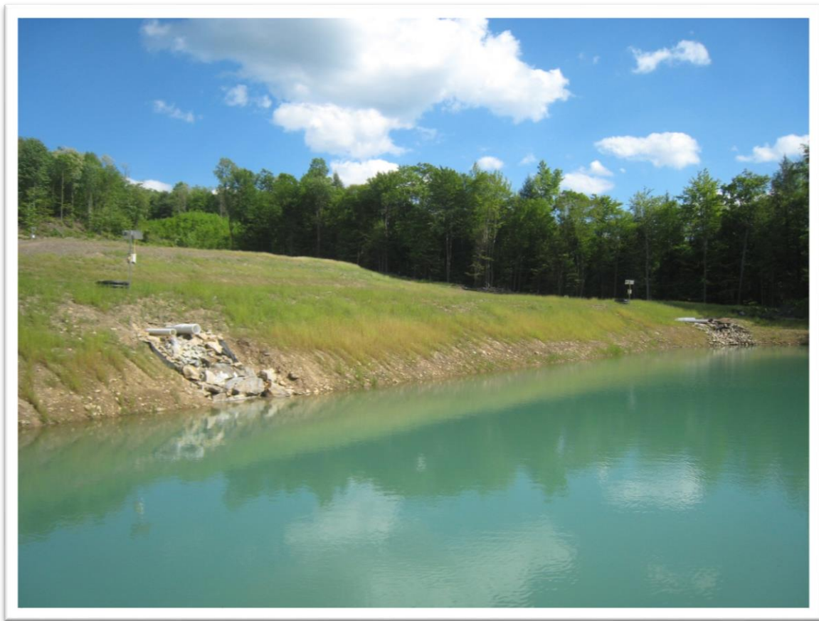
Photo of the settling pond for the upslope limestone ponds in the Gibson Halstock treatment system.
