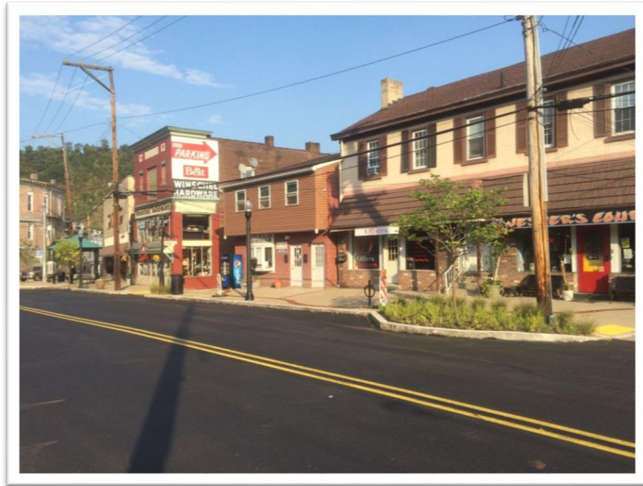
A photo of a street in Etna Borough, recently benefitting from green infrastructure improvements.
