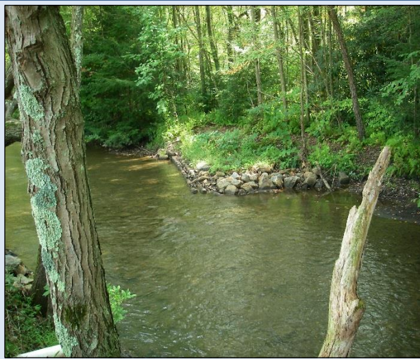
A Log Framed Stone Deflector (left) and a Plunge Pool (right) constructed as part of this volunteer-led habitat improvement project. The installation of these BMPs would have been futile had it not been for the dedicated NPS reduction efforts focused on this watershed years prior.
