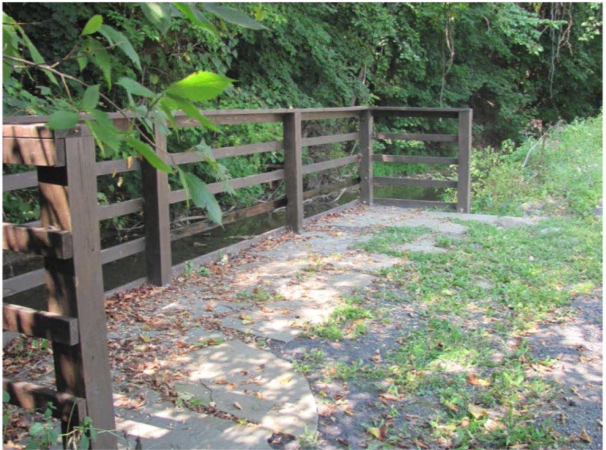
A photo of a platform constructed as part of Project 1315; this platform enhances experiential and environmental education activities.
