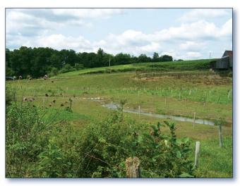
Figure 1. Watershed partners restored this section of Pennsylvania's Pierceville Run by grading streambanks, planting a riparian forest buffer and installing fences to prevent cattle access.
