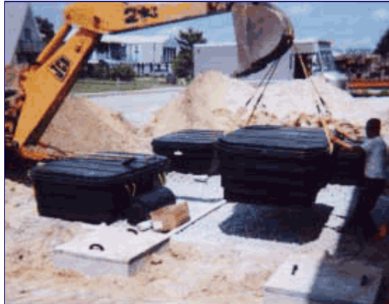
Four Puraflo Units Being Installed
