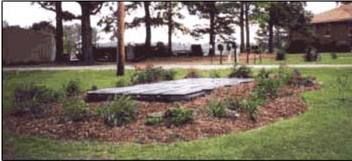
Installed Puraflo peat filter
