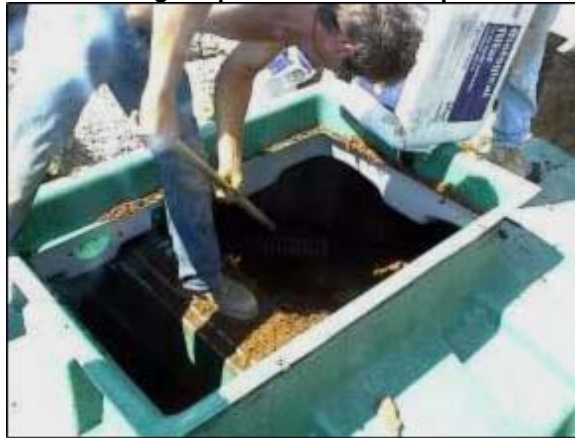
Filling the peat filter with new peat
