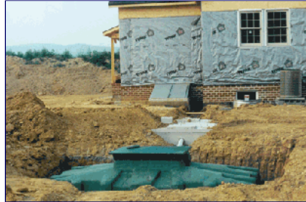
Ecoflo Filter Installation
