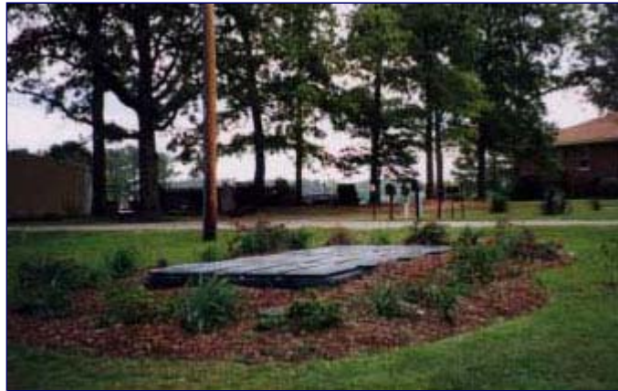
A Completed Seeding and Grading Around Puraflo Filters
