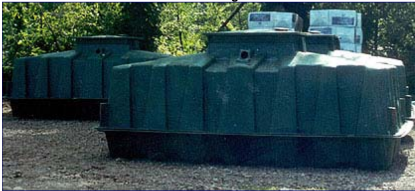
Two Ecoflo Filter Tanks With Bags of Peat to be Installed
