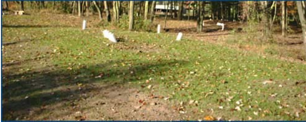
This picture shows an Option A at-grade absorption area that has been seeded. The inspection ports and lysimeters are for research purposes.
