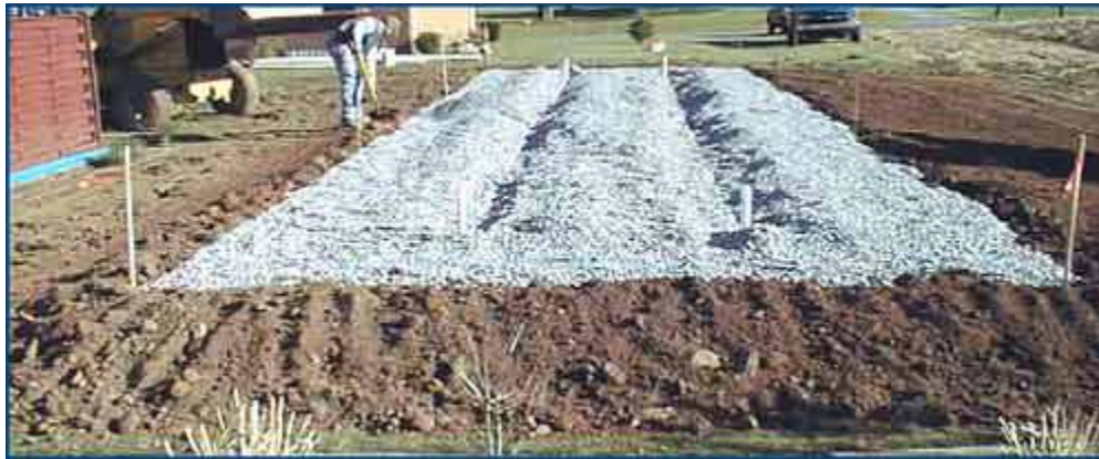
Alternate at-grade absorption area with the distribution pipes installed.
