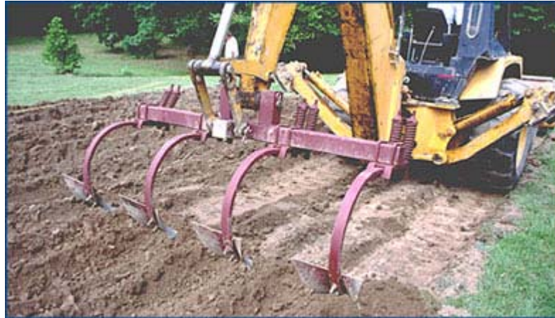
An alternate at-grade absorption area being chisel plowed.
