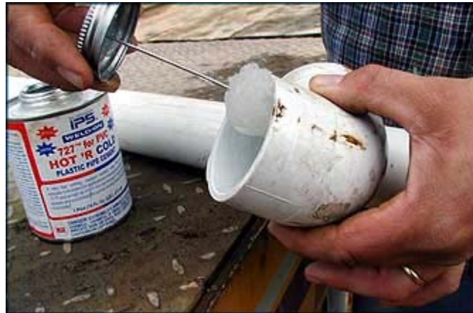
Pipes being glued
