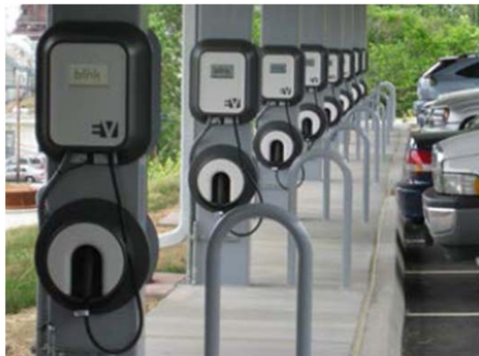
Figure 10 – Level II Fleet Charging Stations
