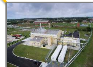
CHP Plant 3.5 MW / 60 kpph Capacity
