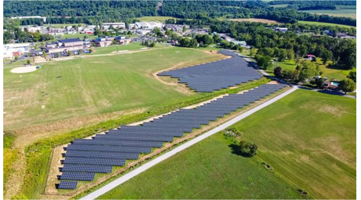
Behind the High School 2.1 MW Bifacial panels
