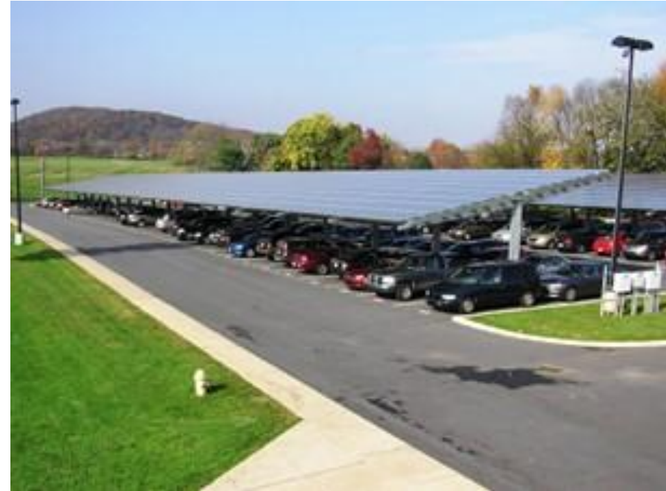
Solar Parking Canopy at Freedom High School
