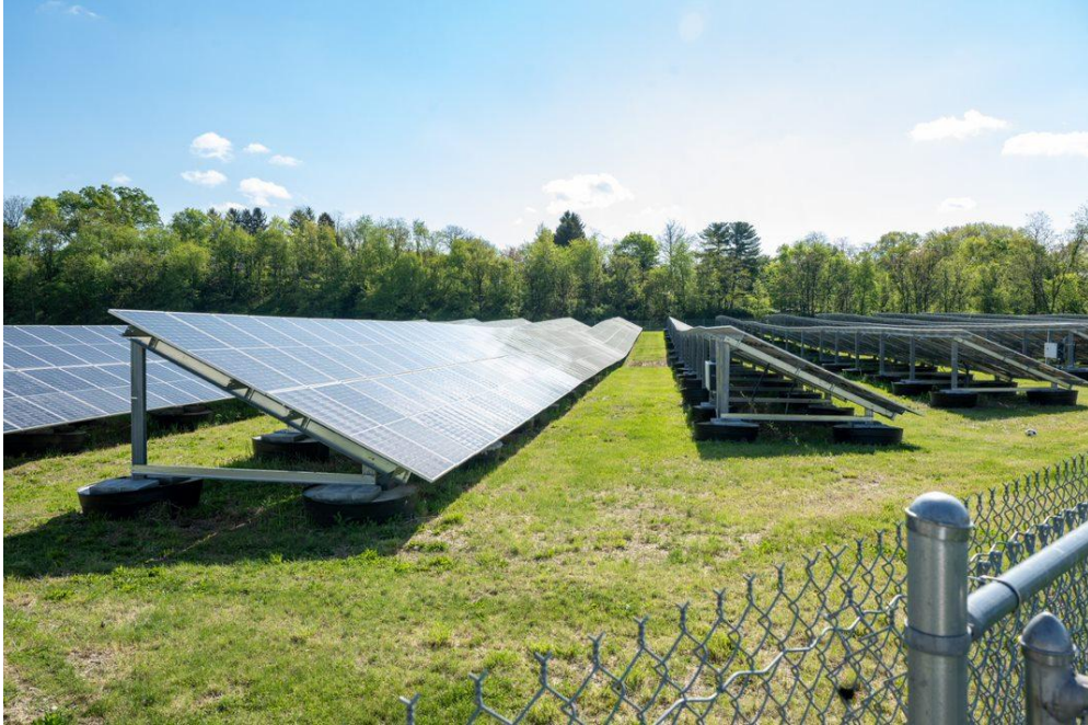
Typical ground mounting system with perimeter fencing
