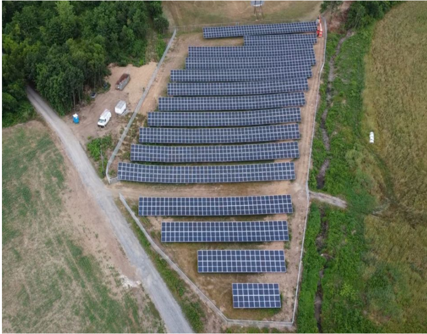
West Snyder Elementary School 460KW
