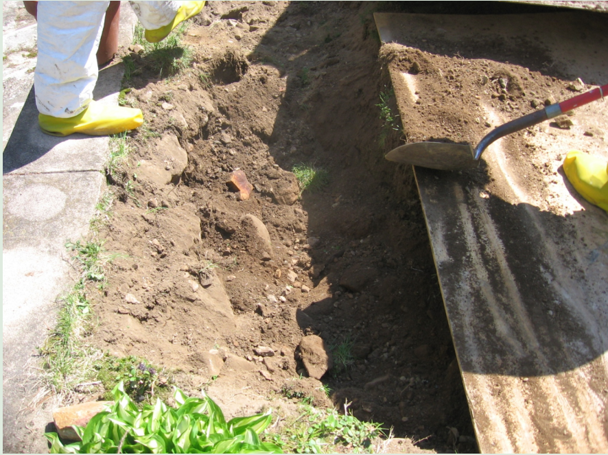
Personal protective outerwear was required to remediate battery casing material intermingled with soil, cobbles and other fill material at the Mt. Laurel Battery Casing Site, Alsace Township, Berks County, Pennsylvania.
