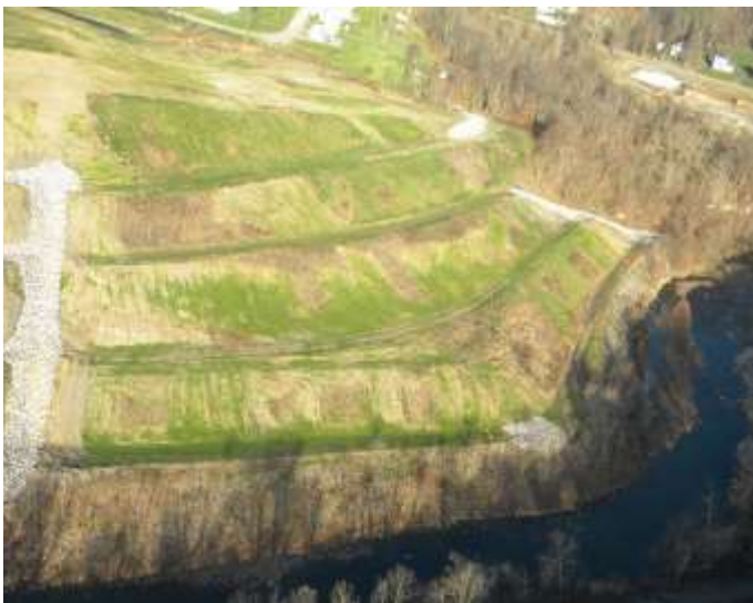
Terraced face and stormwater controls above creek.
