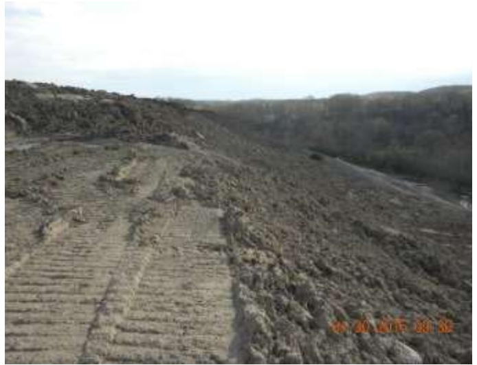
Grading of soil covering material on terraced face above creek facing northeast.
