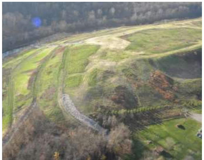
Terraced face and stormwater controls above creek.
