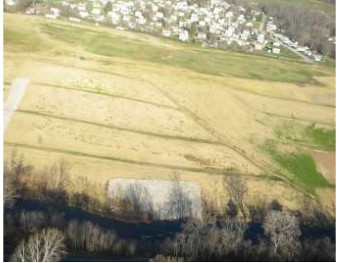
Terraced face, stormwater controls above creek and rock armoring.
