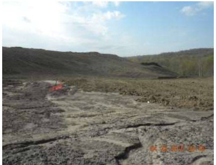
Grading of soil covering material along southern face.
