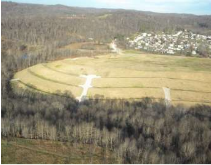
Terraced face and stormwater controls above creek.
