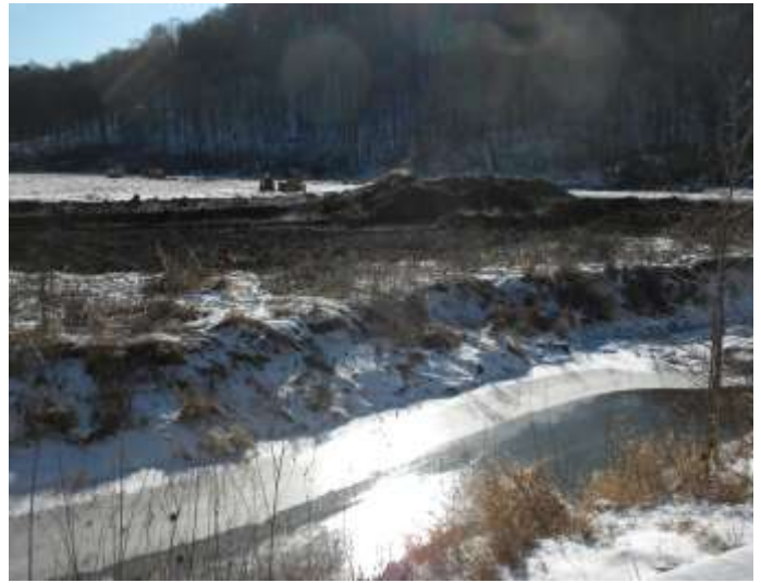
Excavated soil material.
