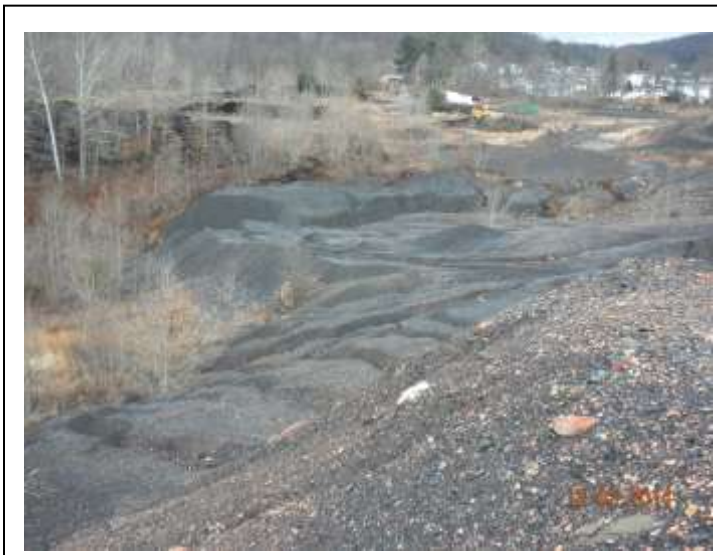
Base of pile of its southern face.
