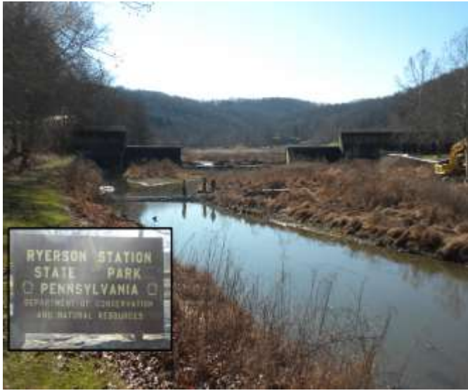
Outside face of dam.
