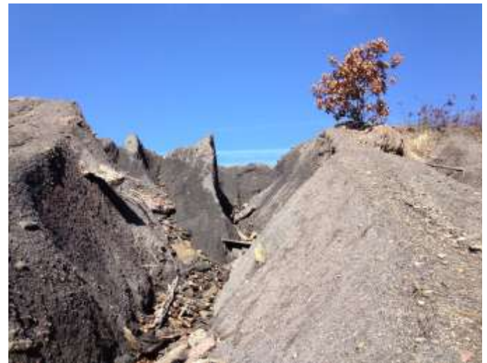
Typical eroded refuse gorge.
