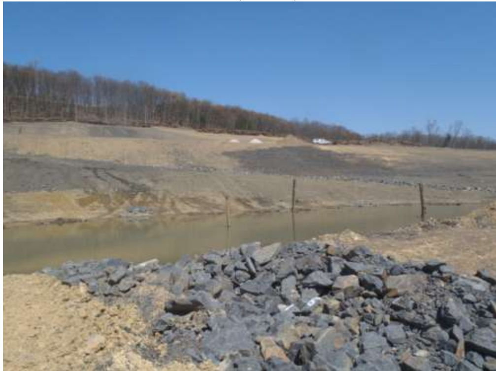
Grading Area 'D' during construction
