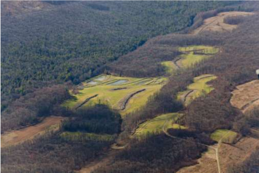
Oblique showing completed job first fall.
