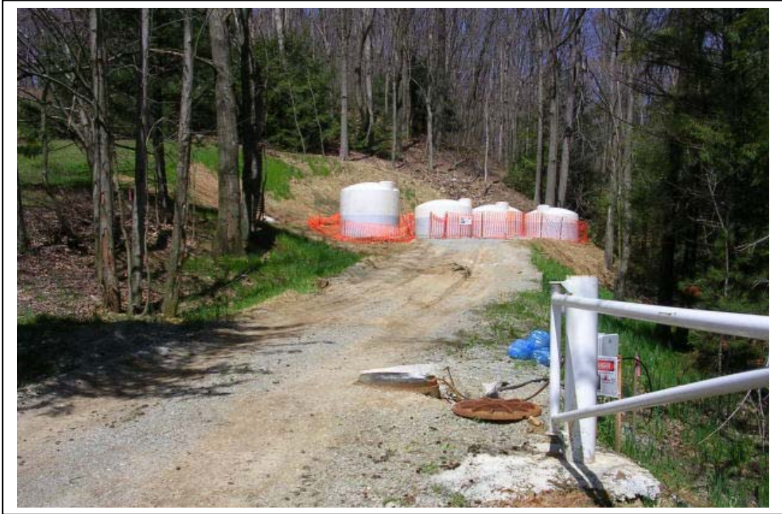
Mine pool dewatering and chemical treatment at Melcroft #1 Mine (Kalp site)
