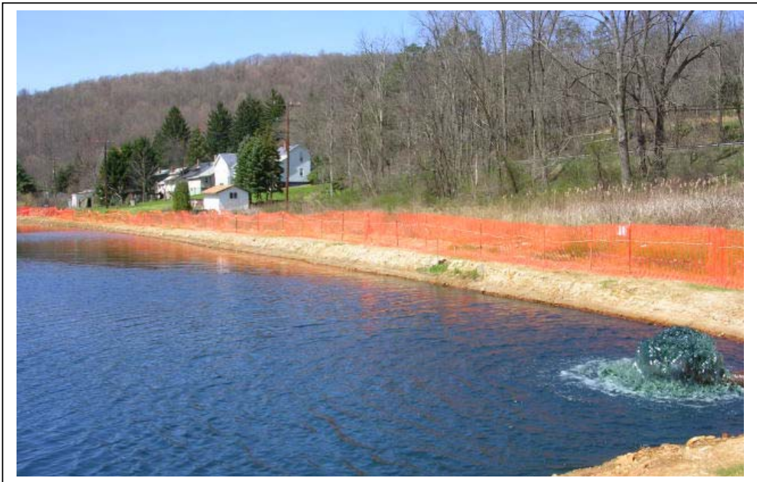
Mine pool dewatering and chemical treatment at Melcroft #1 Mine (Kalp site)
