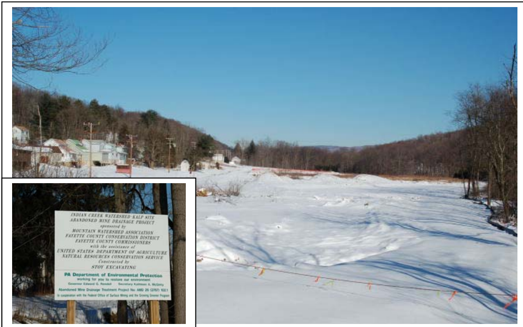
Passive treatment construction area at the Kalp site
