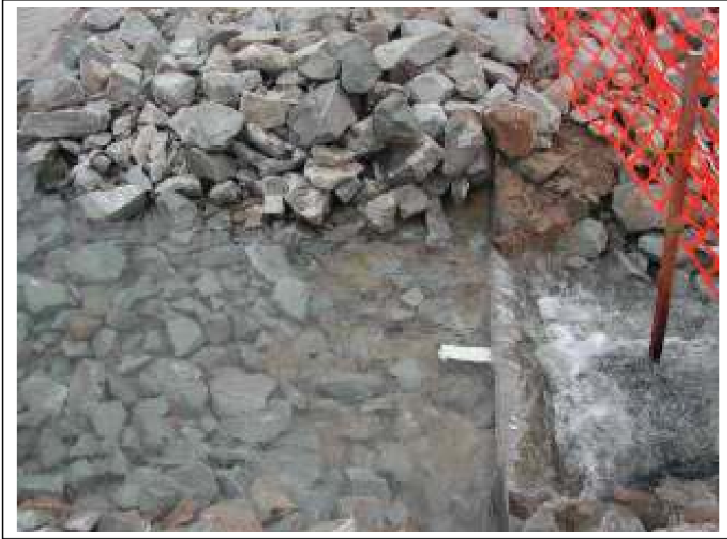
Treated discharge during mine pool dewatering
