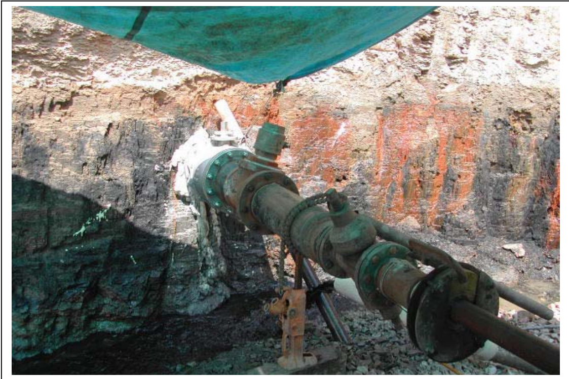
Directional Drilling at Melcroft #3 Mine (Melcroft site)
