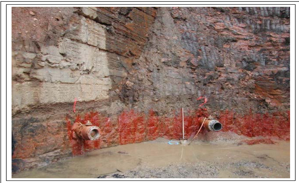
Completed Directional boreholes at Melcroft #3 Mine (Melcroft site)
