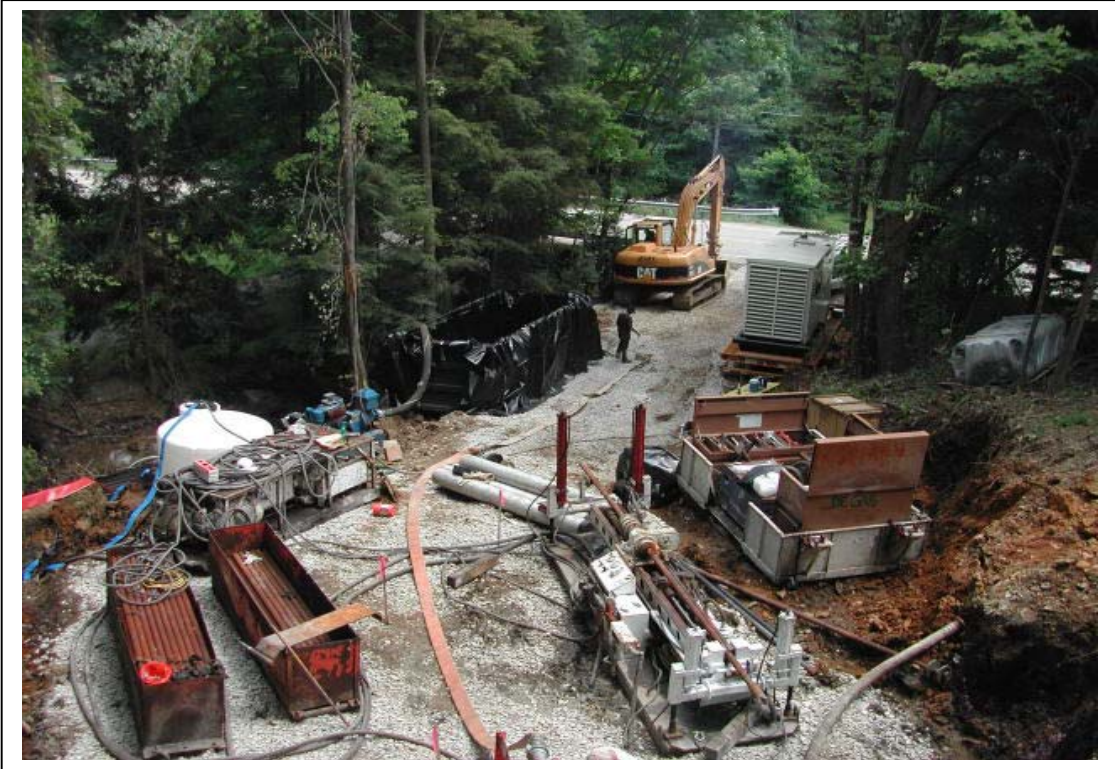
Directional drilling at Melcroft #1 Mine (Kalp site)
