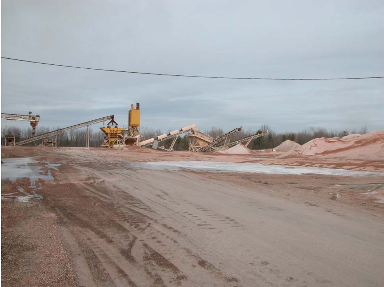
Figure 3.7. Coal ash conveyor at left of photo delivers ash from Gilberton Power Company FBC plant to mineral processing equipment shown in center of photo to produce an aggregate which meets PA Department of Transportation specifications.
