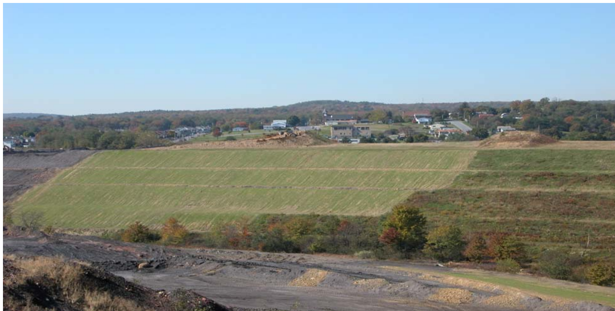
Figure 5.1. Photograph of the reclaimed portions of the Revloc 1 refuse site. Note the contrast with Figure 5.2.
