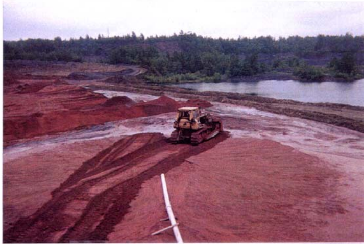
Figure 7.10. A D8 operating on the surface of the slurry-placed ash after closure of the demonstration pond.
