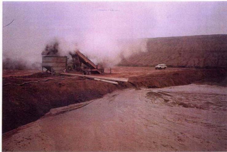
Figure 7.9. Photograph of the slurry placement facility.
