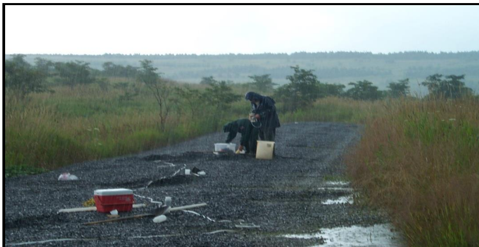
Figure 7.3. Typical Manganese Removal Bed
