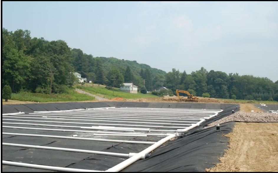
Figure 7.9. Limestone being placed on top of the underdrain piping system
