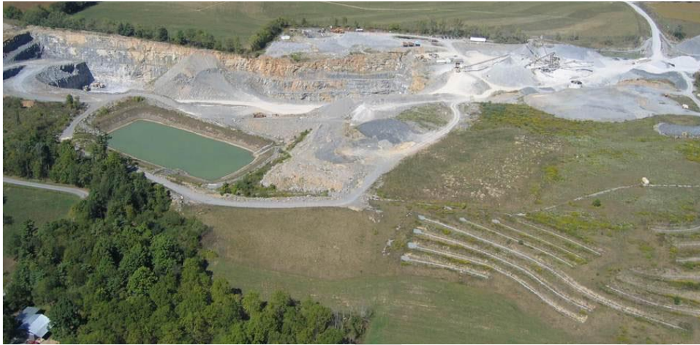
Figure 5.7. Limestone Quarry Subsurface Infiltration Gallery and Pond (Aerial View)
