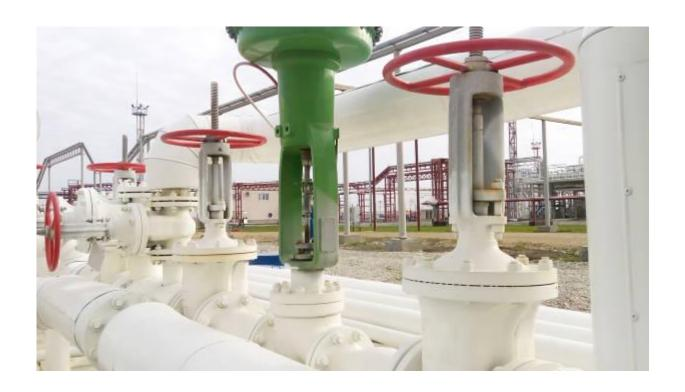
green pneumatic pump valve on the pipeline
