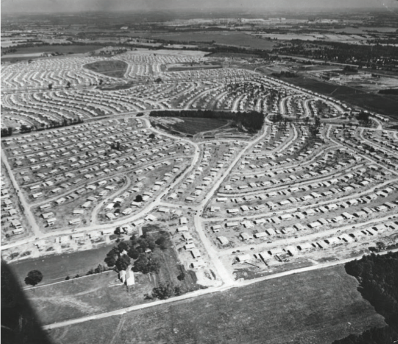
Figure 4.2 Aerial view of Levittown, 1952. (Courtesy: Temple University Libraries, Special Collections Research Center, McDowell Evening Bulletin Collection.)
