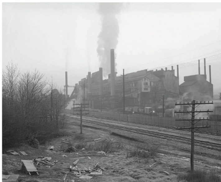
Figure 5.3 New Jersey Zinc Company, Palmerton Plant, Carbon County, Pennsylvania. Placed on the Superfund program's National Priorities List in 1983. (Courtesy: Library of Congress, Historic American Engineering Record.)
