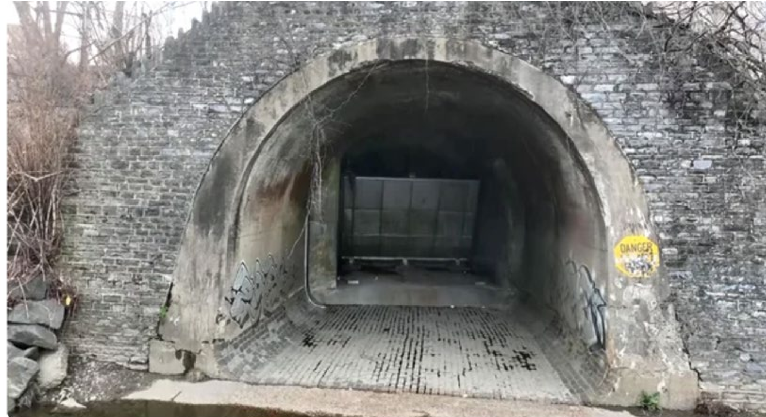
Outfall T14, located along the confluence of Frankford and Tacony Creek, is the city's largest outfall. Nearly 2 billion gallons of raw sewage and polluted stormwater flowed out of T14 between July 2023 and June 2024.
