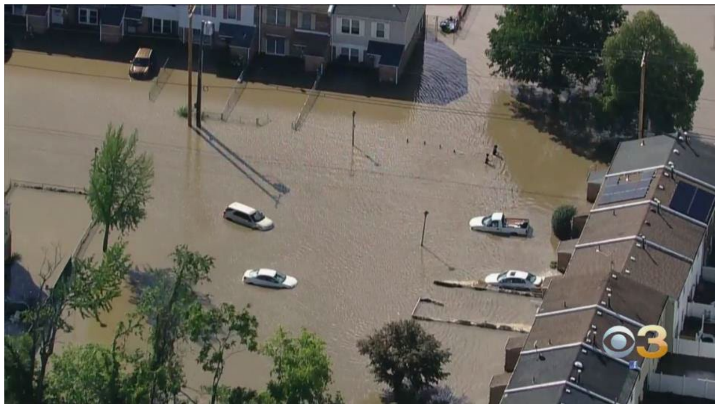
Flooding in Eastwick, Philadelphia from Tropical Storm Isaias
