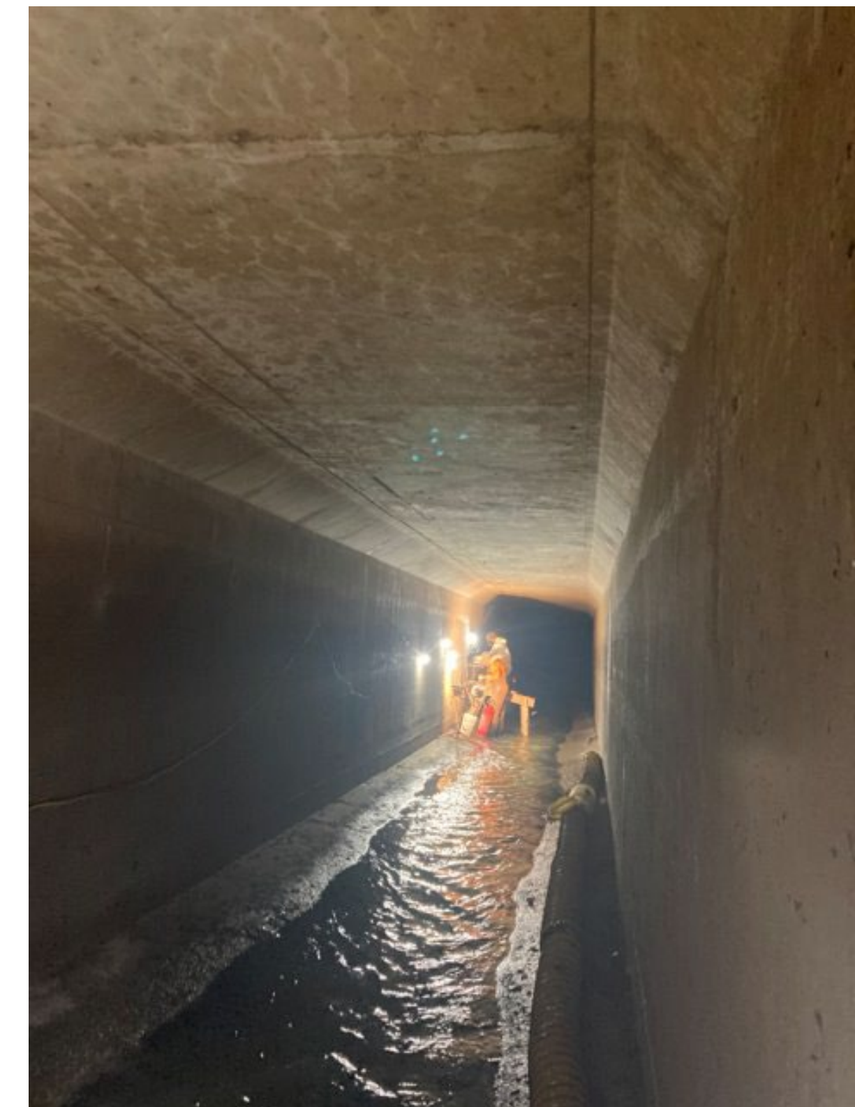
Tacony Creek Interceptor Rehab/Lining
