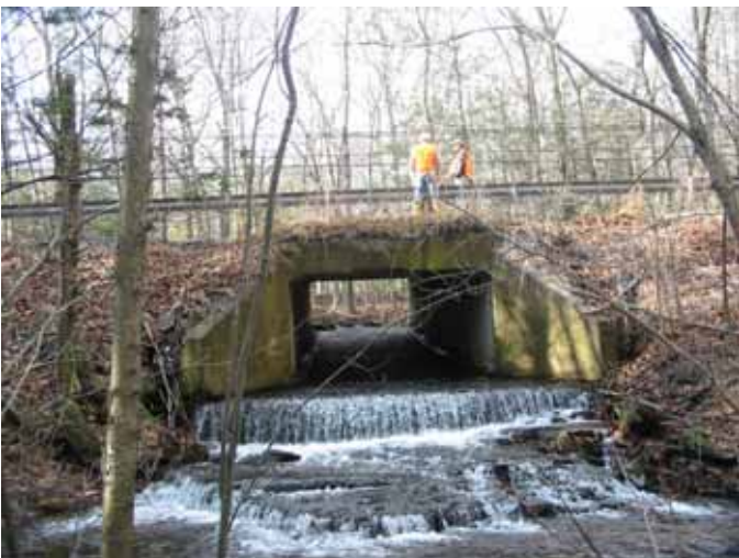
Figure 9 - Cranberry Creek at Route 191 crossing. This location receives a large quantity of road runoff, which should be managed to reduce introduction of pollutants to stream.
