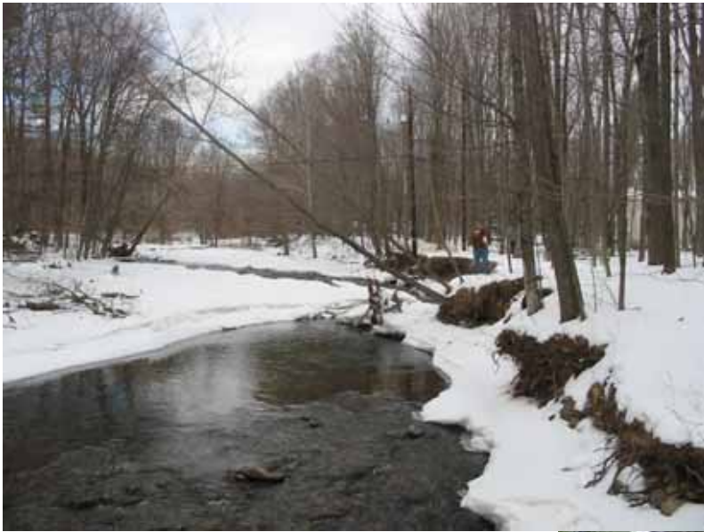
Figure 19 – Upper Paradise Project 1: Paradise Creek from the vicinity of Red Rock Road to Lake Crawford. Previously channelized, this reach is now widening, forming meanders, and threatening private property. Note the telephone pole in background, once about 15 feet from the stream, is now about to be undermined. A more detailed assessment and restoration is recommended from Red Rock Road to Lake Crawford.
