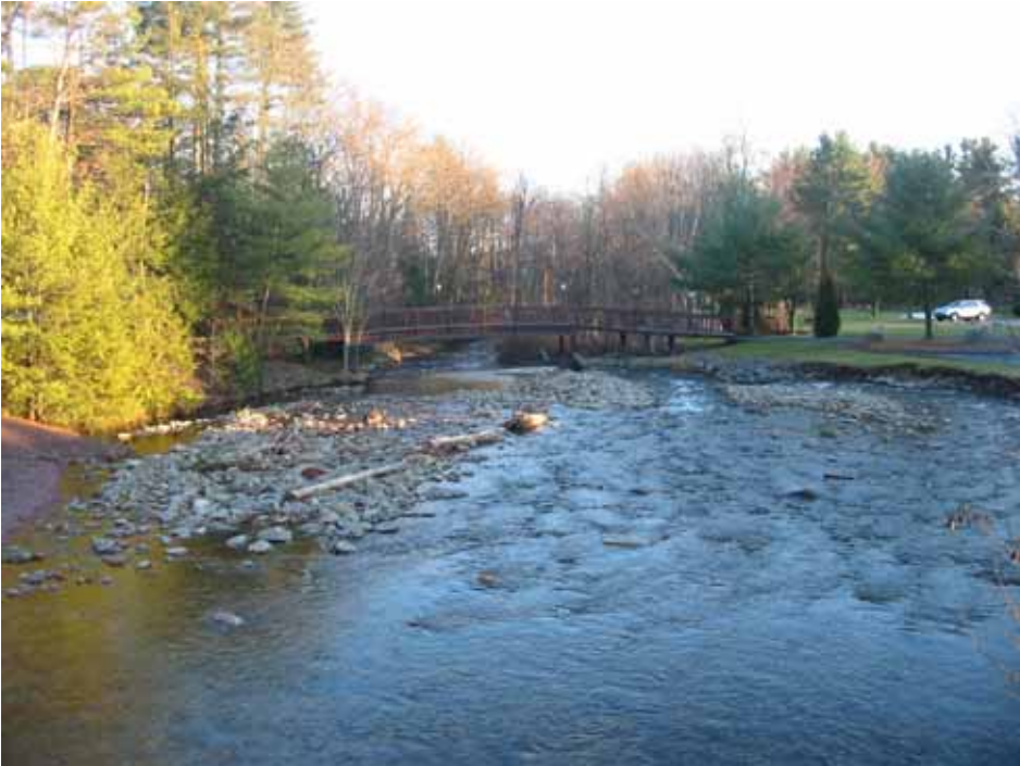
Figure 24 - Downstream view of sediment-filled small impoundment on Devils Hole Creek. The dam is just upstream of the footbridge in the background, and is located about 100 yards upstream of the confluence of Devils Hole Creek and Paradise Creek. Bank erosion to the right threatens a driveway and building. Dam removal is recommended at this location. Unless such impoundments are maintained frequently, installation of dams in high-energy stream environments is discouraged.
