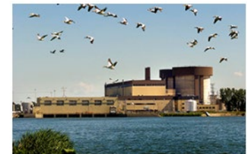
Braidwood Generating Station
