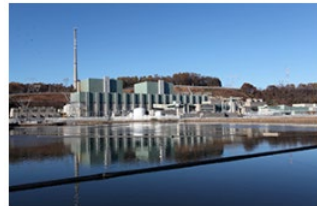
Peach Bottom Atomic Power Station
