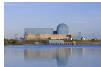
Clinton Power Station
