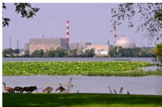
Dresden Generating Station
