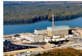
Quad Cities Generating Station
