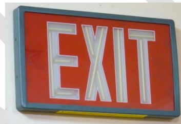
TRITIUM EXIT SIGN
