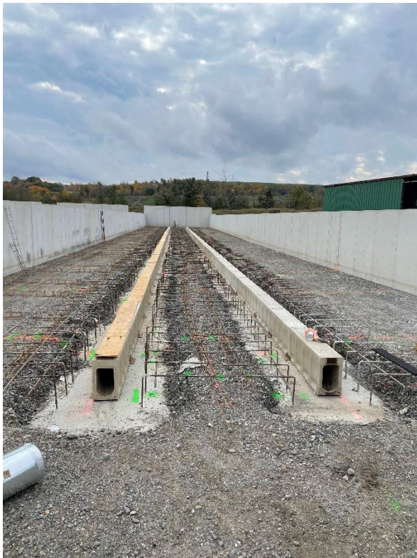
Aeration-Moisture Removal Channel Installation
