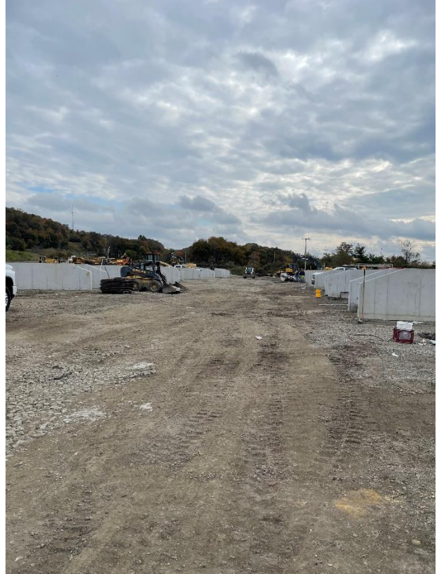
Bunker Construction Looking Down Access Road
