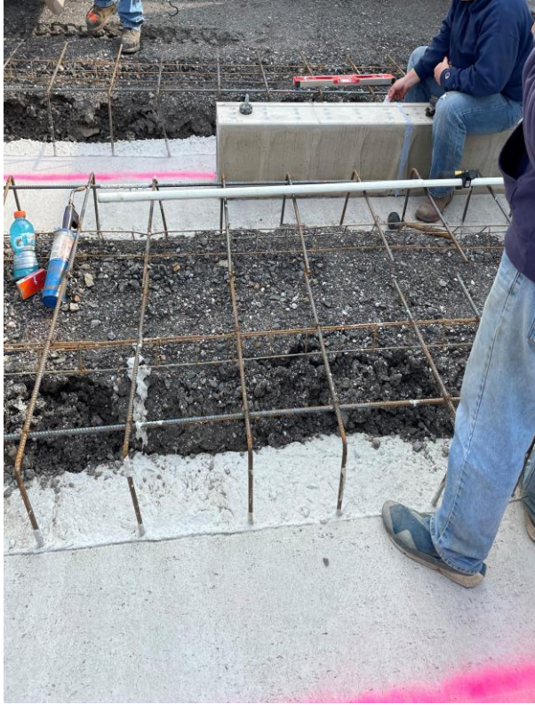
Setting Aeration-Moisture Removal Channels
