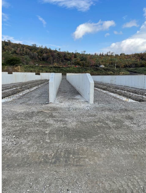
Gap between Bunkers Where Gore Blanket Machine will Operate
