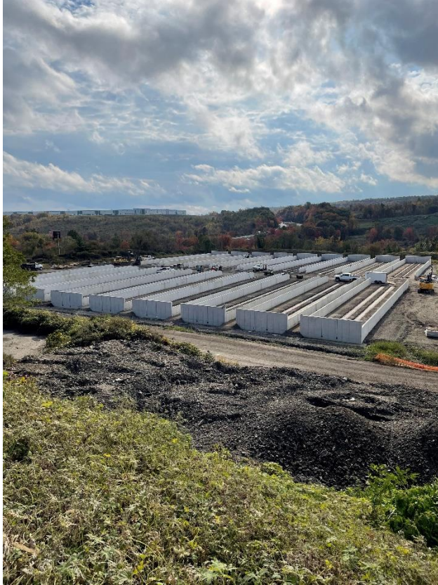
Gore System Bunker Construction 20Oct2023
