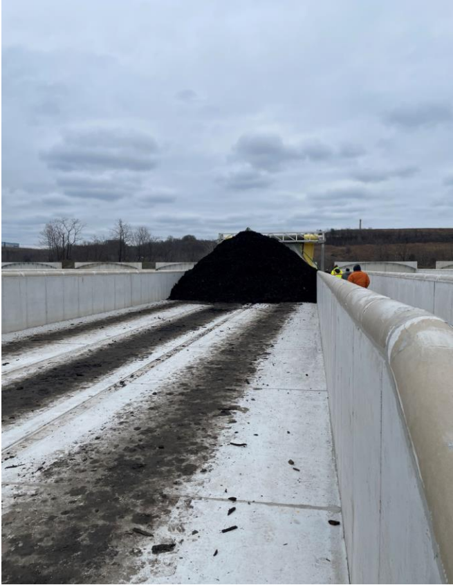
NSP Gore Bunker Partially Filled 5Dec2023
