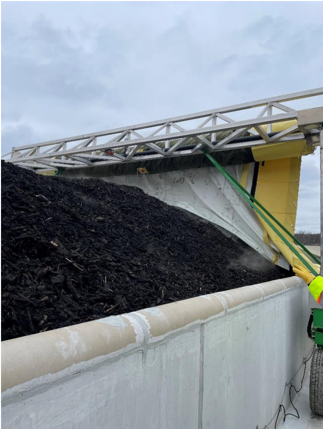
NSP Gore Bunker Partially Covered 5Dec2023
