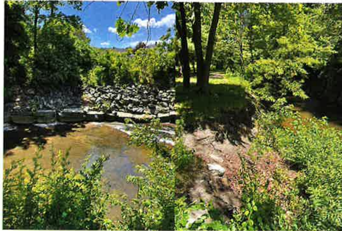
Bank Stabilization Photos
