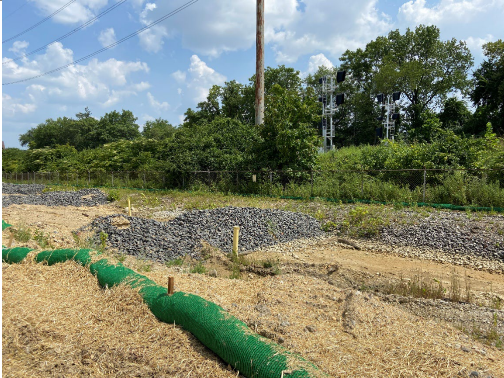
Rock berms and troughs.
