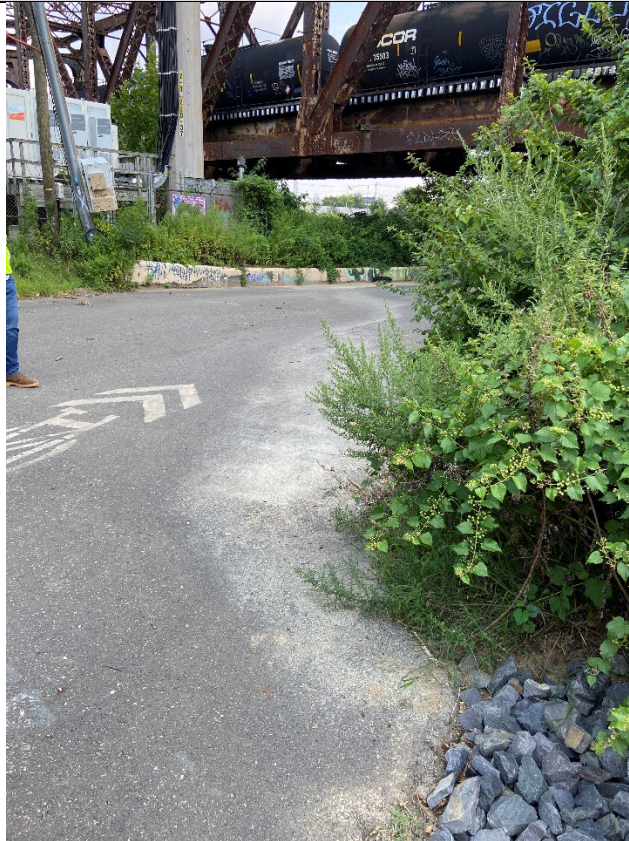
Sediment staining leaving site on to Bartram's Garden trail.
