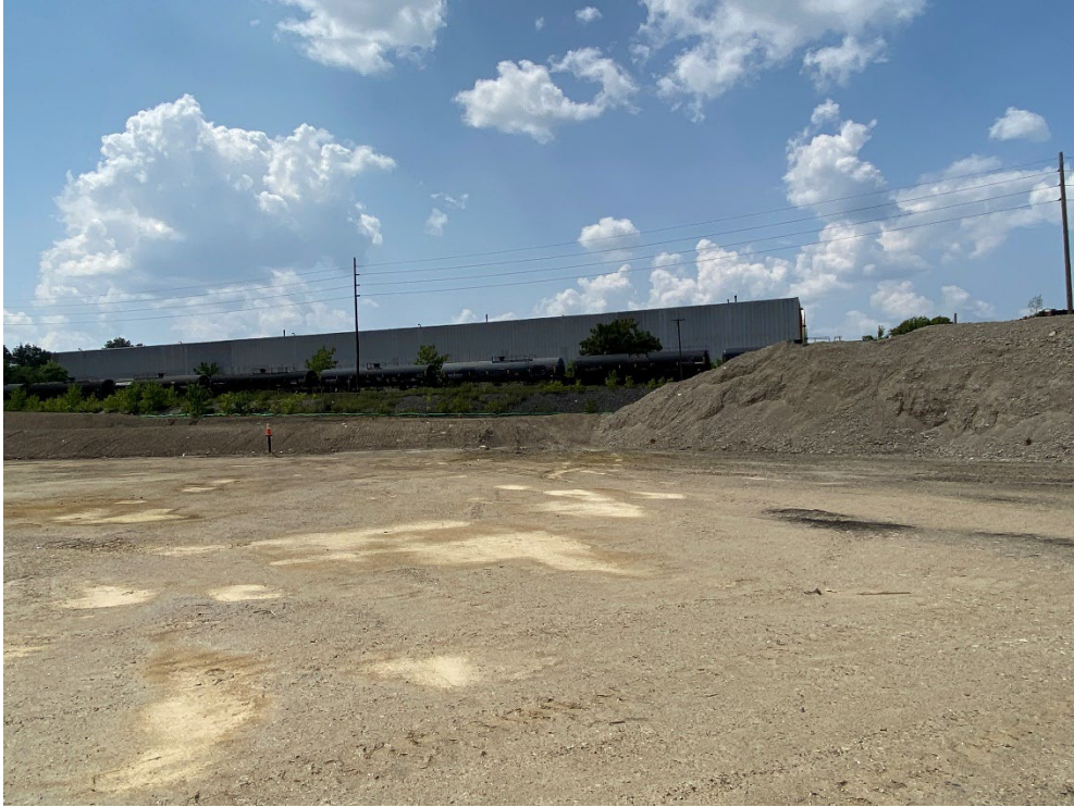
Upslope portion of site.
