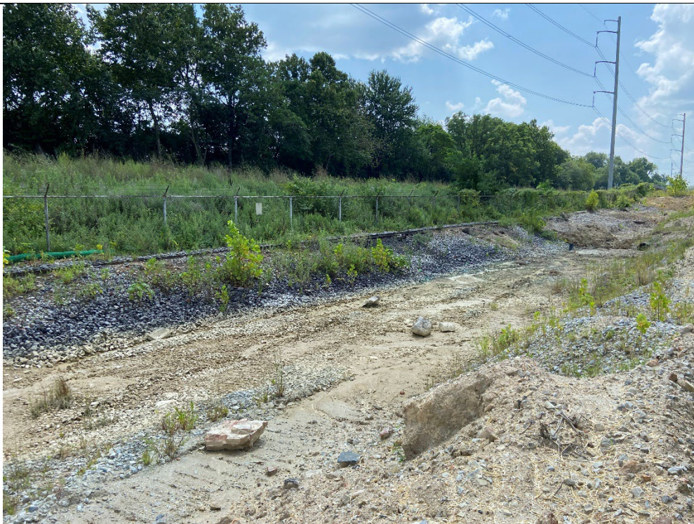
Drainage area, upslope of first rock berm, along railroad tracks.
