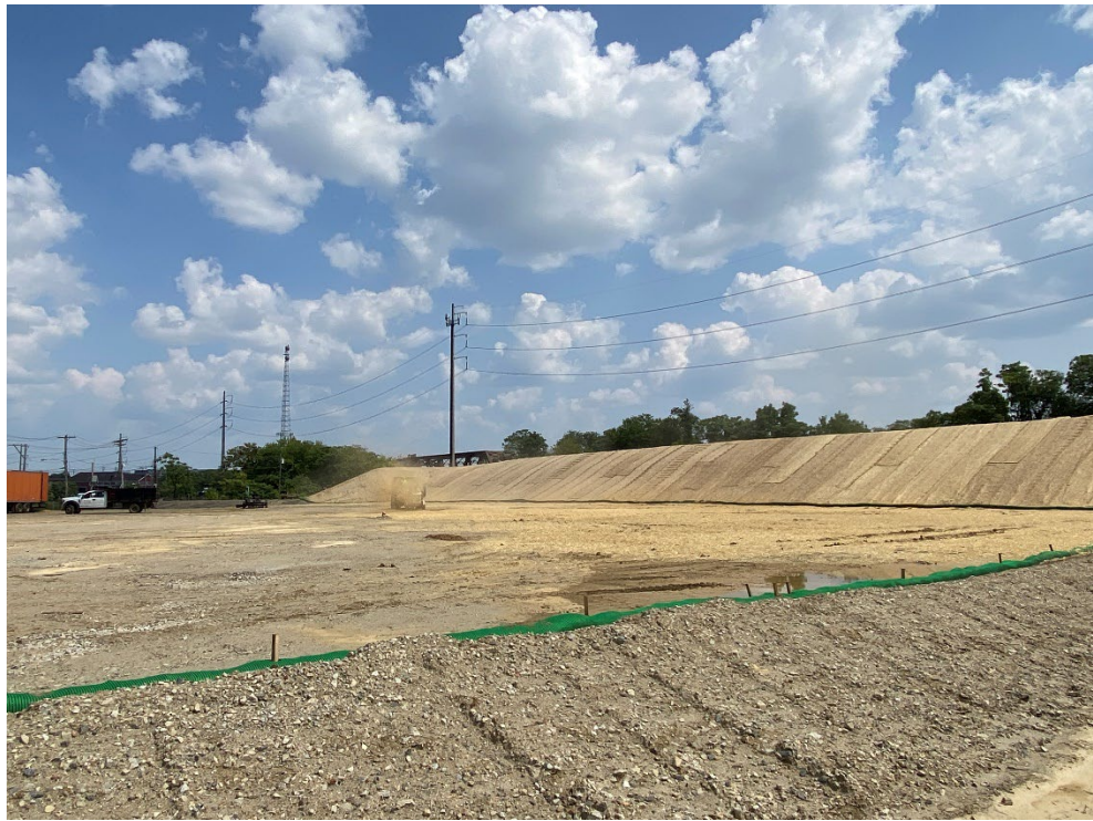
Mulching activity in progress at center.
