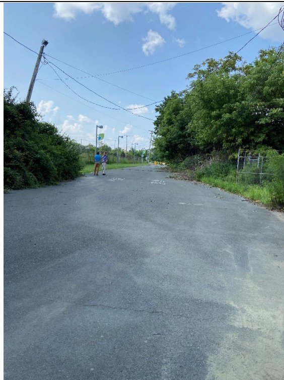
Sediment staining (looking from down-grade to up-grade) on Bartram's Garden trail.
