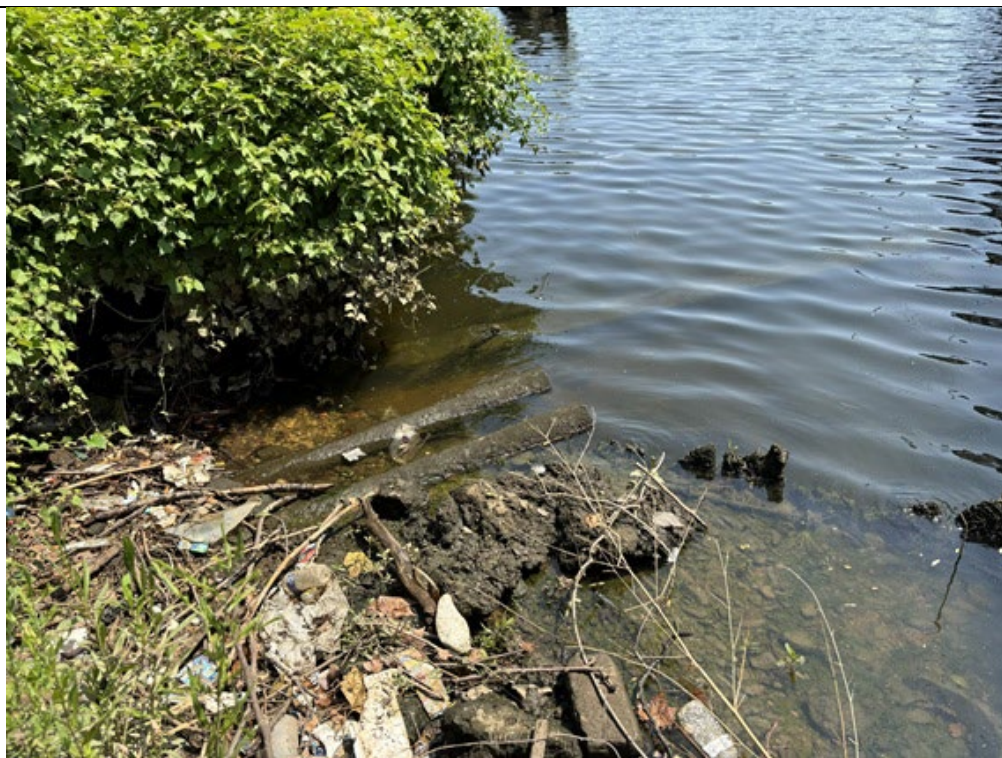
Pipe outfalls (pipes of undetermined origin) across the Bartram's Garden trail from site; half submerged by high tide.
