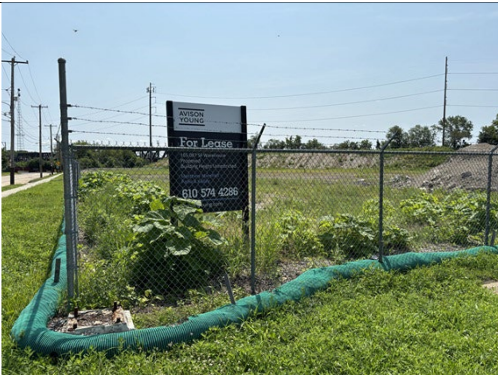
“For Lease signage”, filter sock, and stabilization in midslope portion of site.
