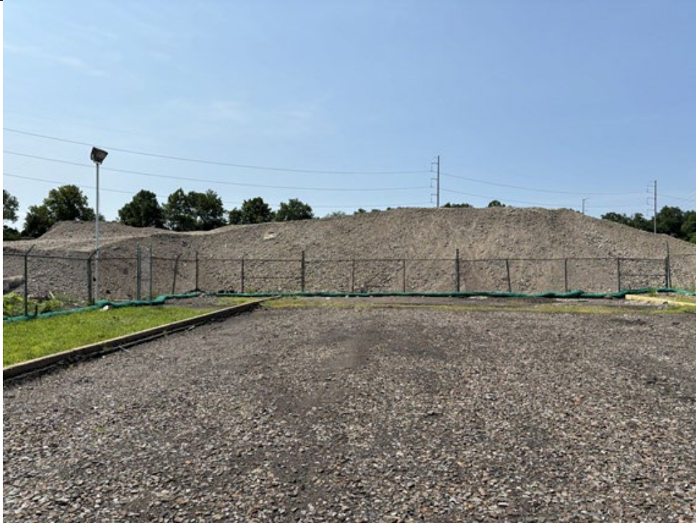
Stone stockpile in midslope section of site.
