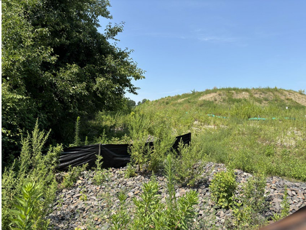
Silt fence and stone lined swale at eastern end of site.
