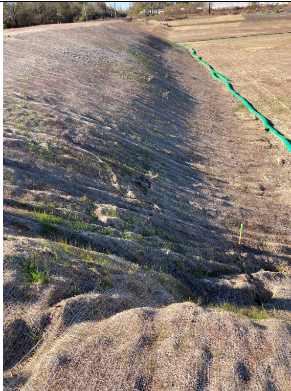
Looking upslope along northern edge of large fill dirt stockpile.
