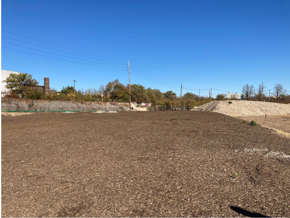
Mulched upslope area, looking towards 51 st St; stone stockpile at right-center.
