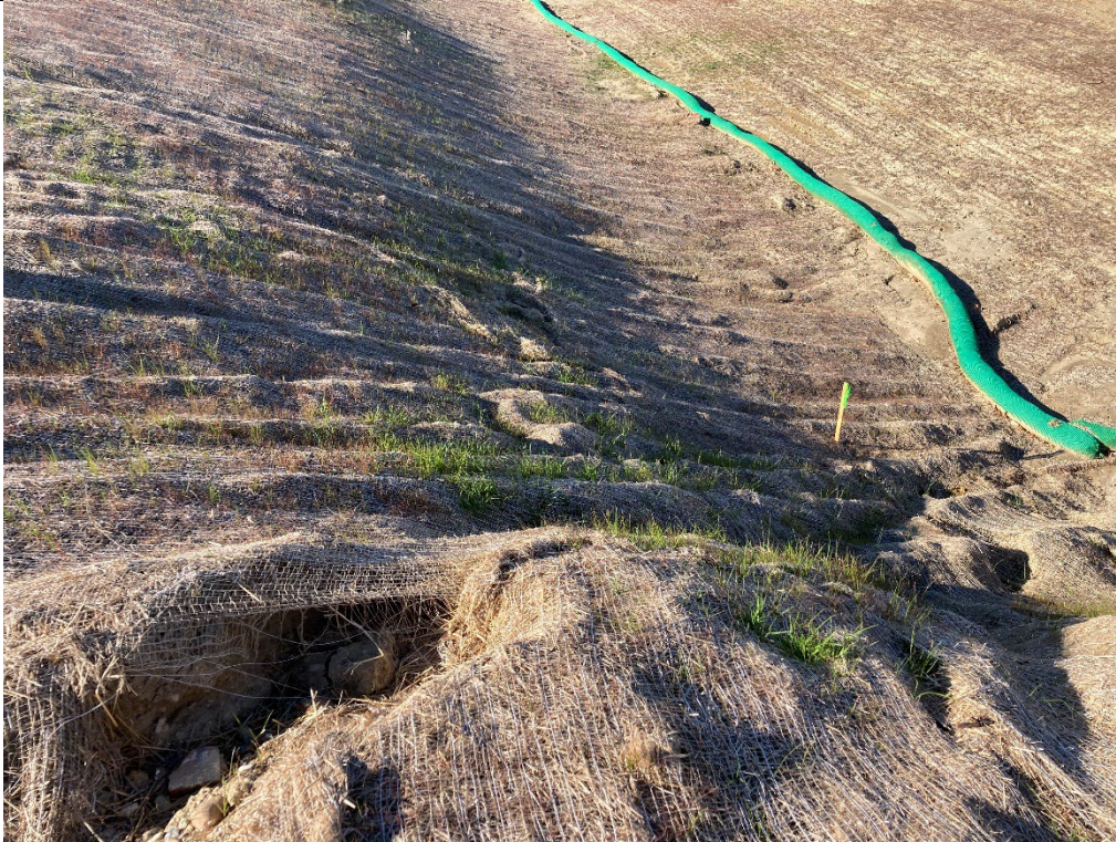
Looking down from top of large fill dirt stockpile with erosion gullies present.
