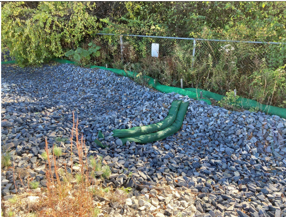
Filtersock intended to capture heavy metals near downslope end of swale.
