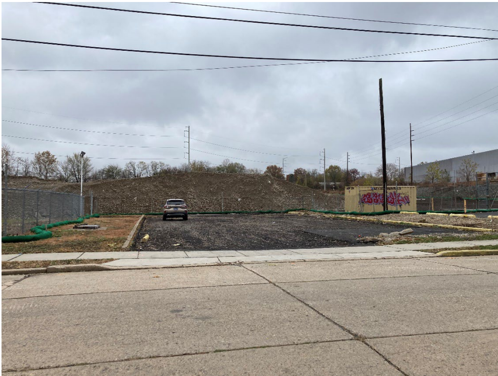
Stone stockpile, taken from 51 st St.
