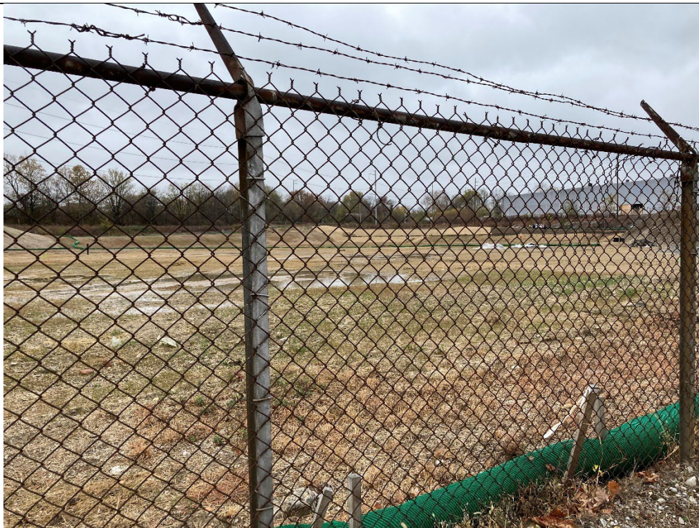
Standing water on middle portion of site after recent rain, looking upslope.
