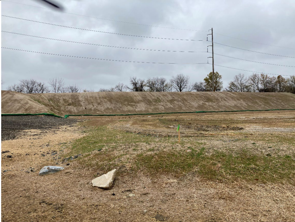
Large fill dirt stockpile.
