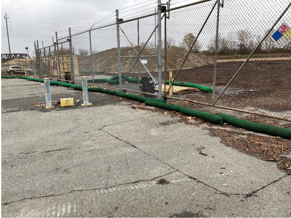
Most upslope gate, along 51 st St.
