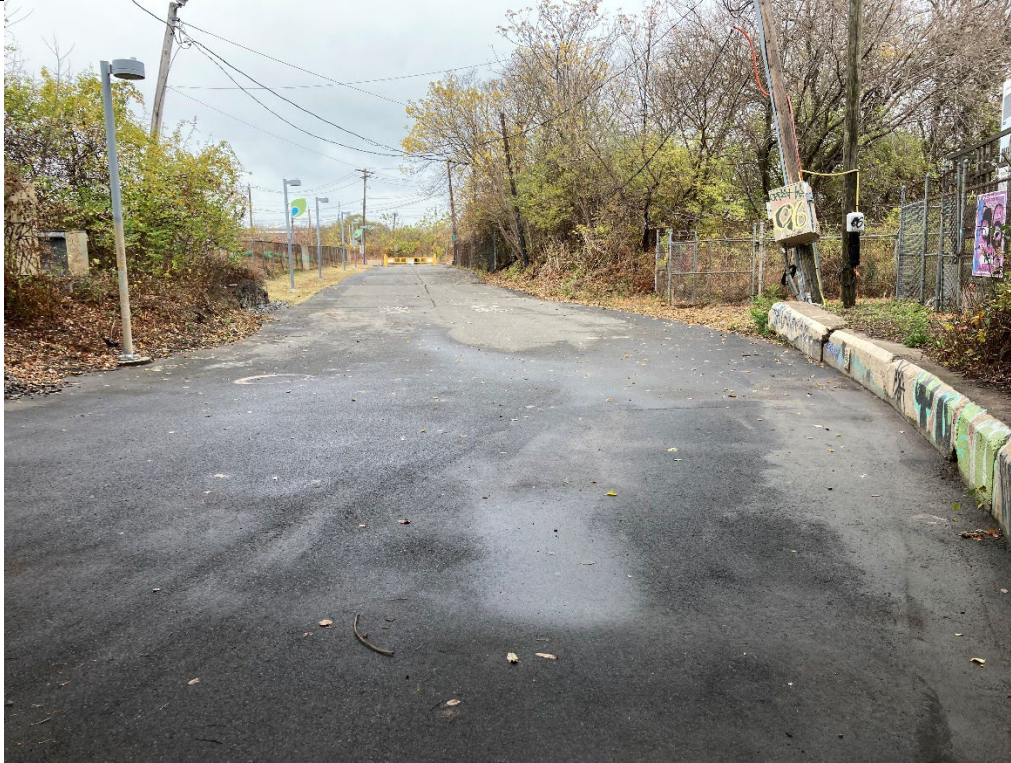
Bartram's Garden trail, taken from under railroad bridge. End of photo log.
