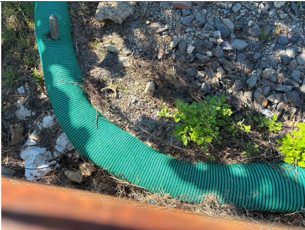
Silt sock at downslope corner of site adjacent to 51 st St. and Botanic Ave.
