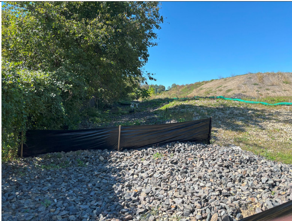
Stone-covered swale and silt fence along railroad tracks.
