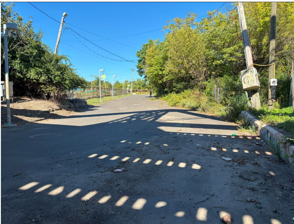
Bartram's Garden trail with pebbles, sediment, and leafy debris under railroad bridge.
