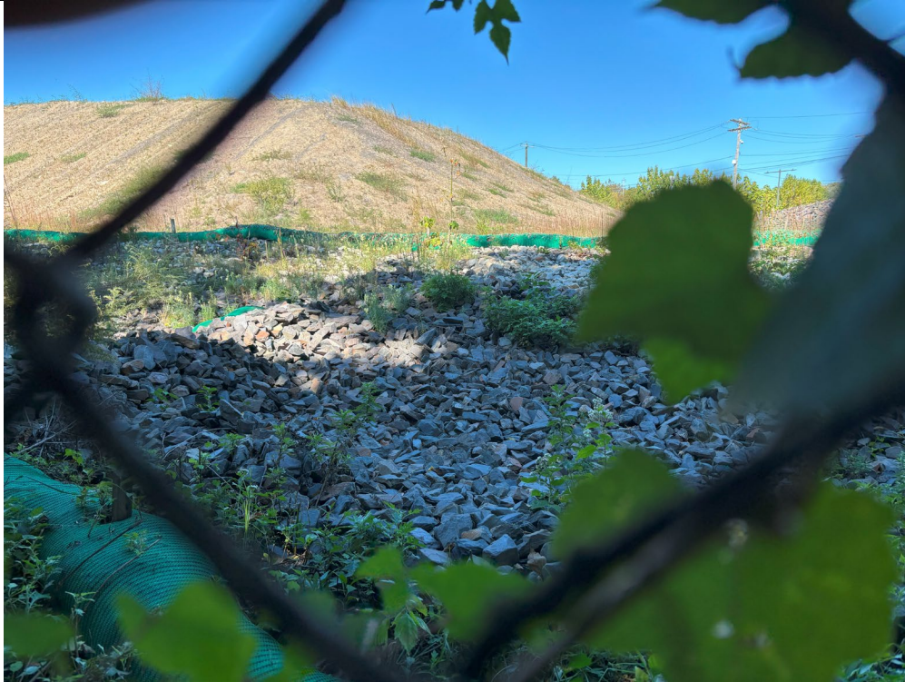
Stone lined swale and downslope end of large fill dirt stockpile from security chainlink fence along railroad tracks.
