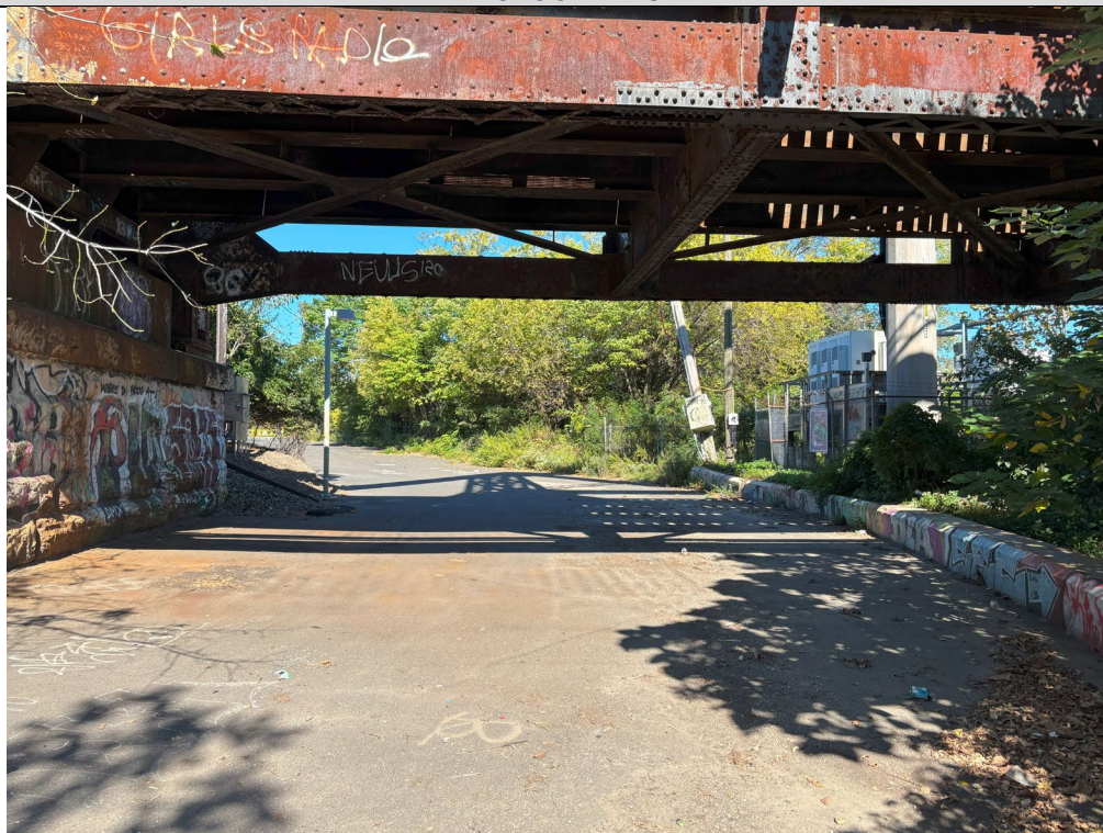
Bartram's Garden trail under railroad bridge.
