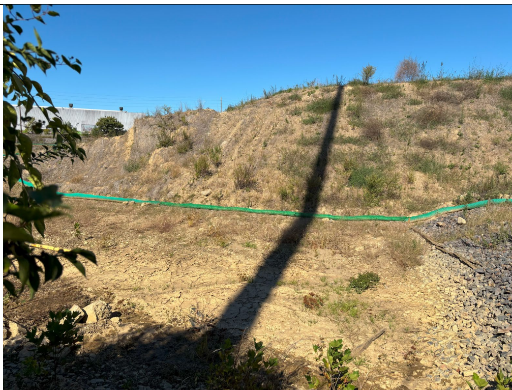
Upslope, back side of large fill dirt stockpile and beginning of stone-lined swale at bottom right.
