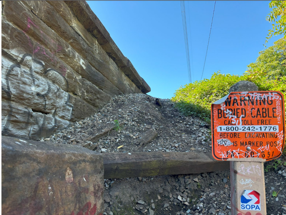
Embankment between railroad tracks (at bridge) and Bartram's Garden trail.
