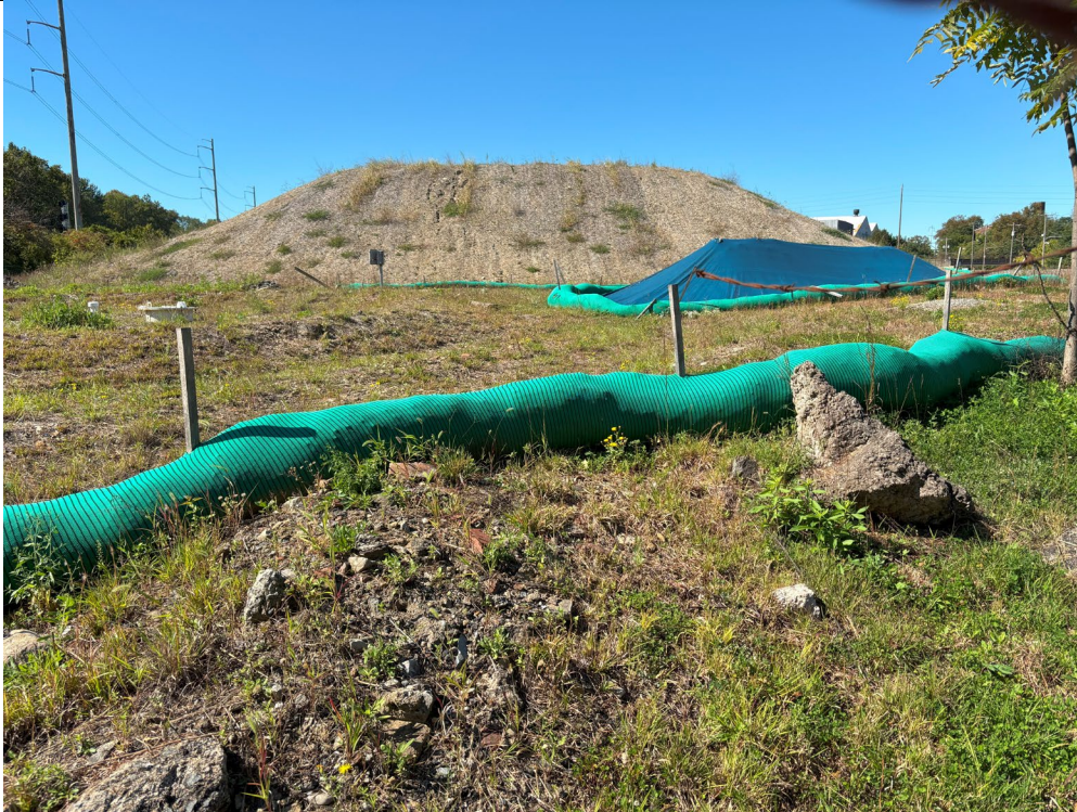
Downslope facing slope of large fill dirt stockpile with covered contaminated fill dirt stockpile in front.
