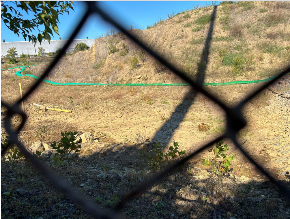
Upslope, back side slope of large fill dirt stockpile, from security chainlink fence along railroad tracks.
