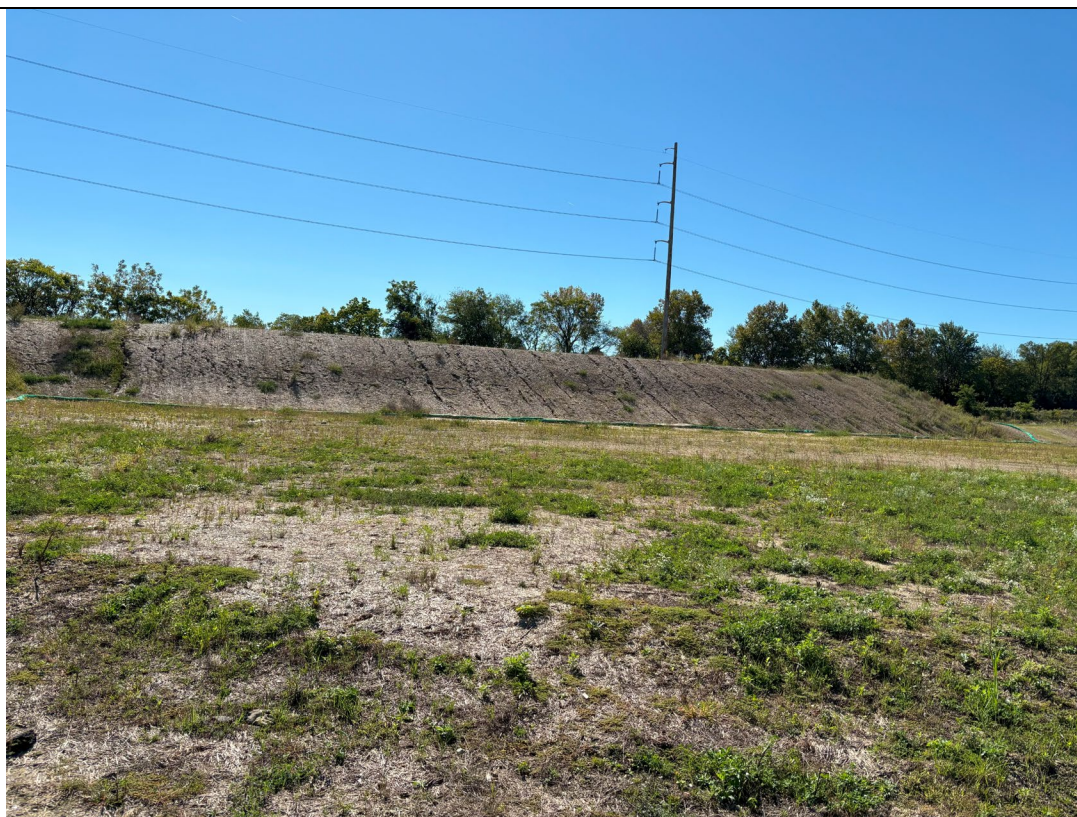
Large fill dirt stockpile in distance with erosions rills and gullies present.
