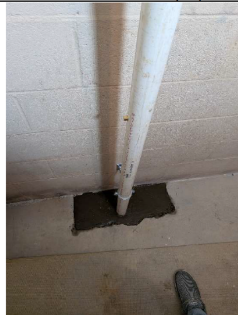
Grout filling opening around vertical extraction point
