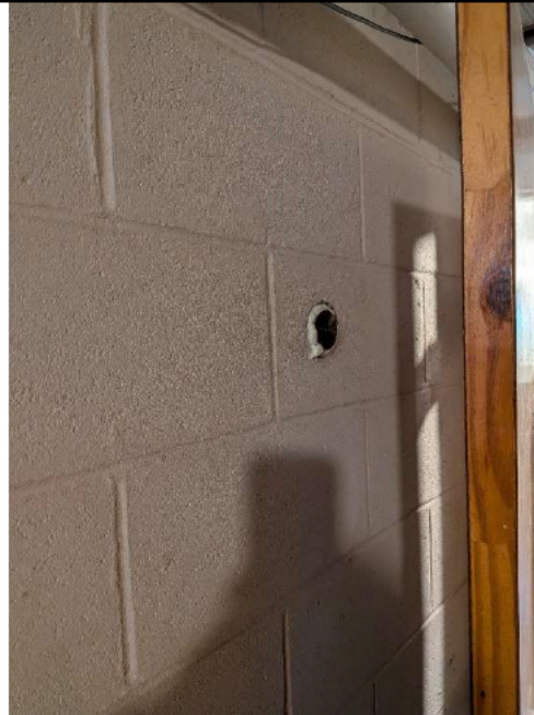
Location of horizontal vapor pin
