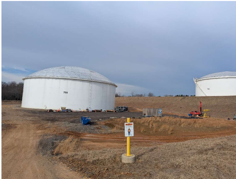
Monitoring well installation in Tank 709 basin
