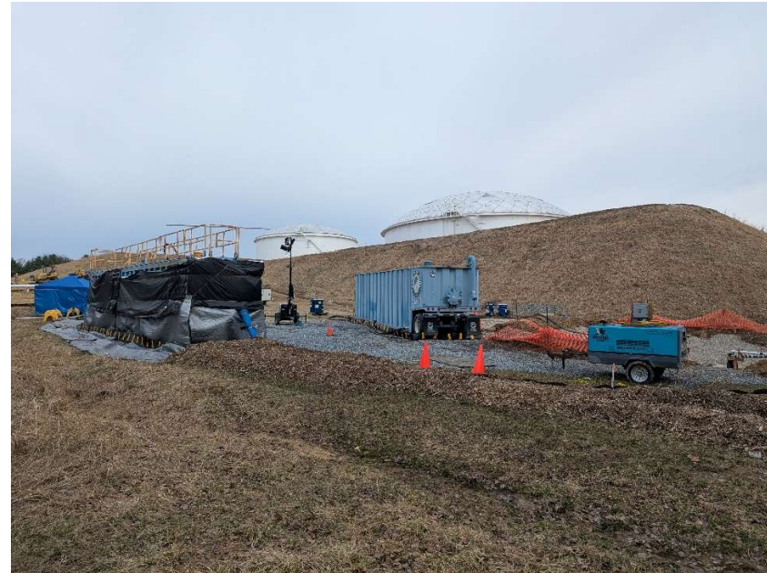
WTU and excavation seep with recovery sump
