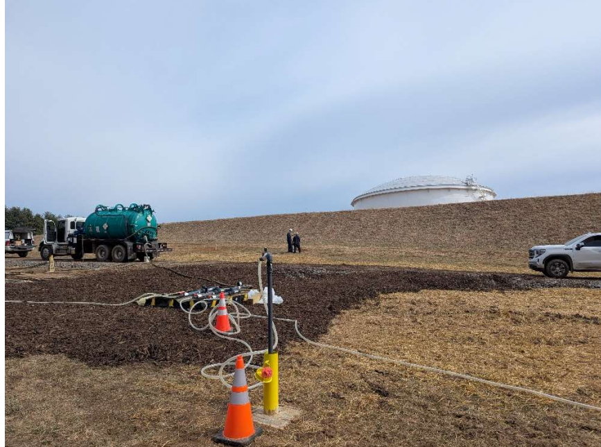
Vacuum truck and effluent located towards the interior of the site
