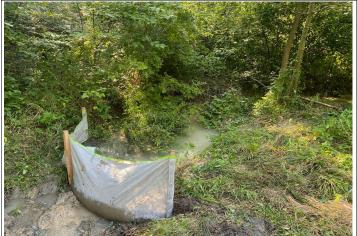
View of sand bag and silt fence dam constructed within stream S-H10 (UNT to Marsh Creek).
