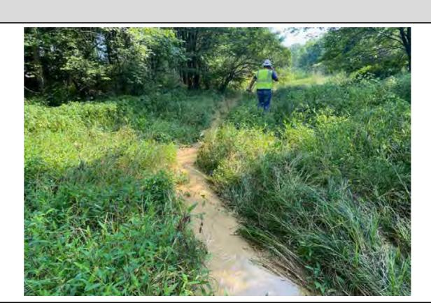
Notes: View of drilling fluid within WL-H17 at location of IR release point.
