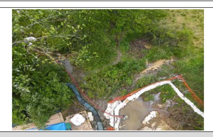
View of contractor personnel using a 4-inch pump to maintain discolored fluid. Fluid remained within existing sand bag containment.
