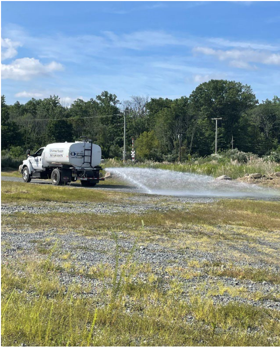
Water truck wetting the roadway- 8/22/23,10:17am
