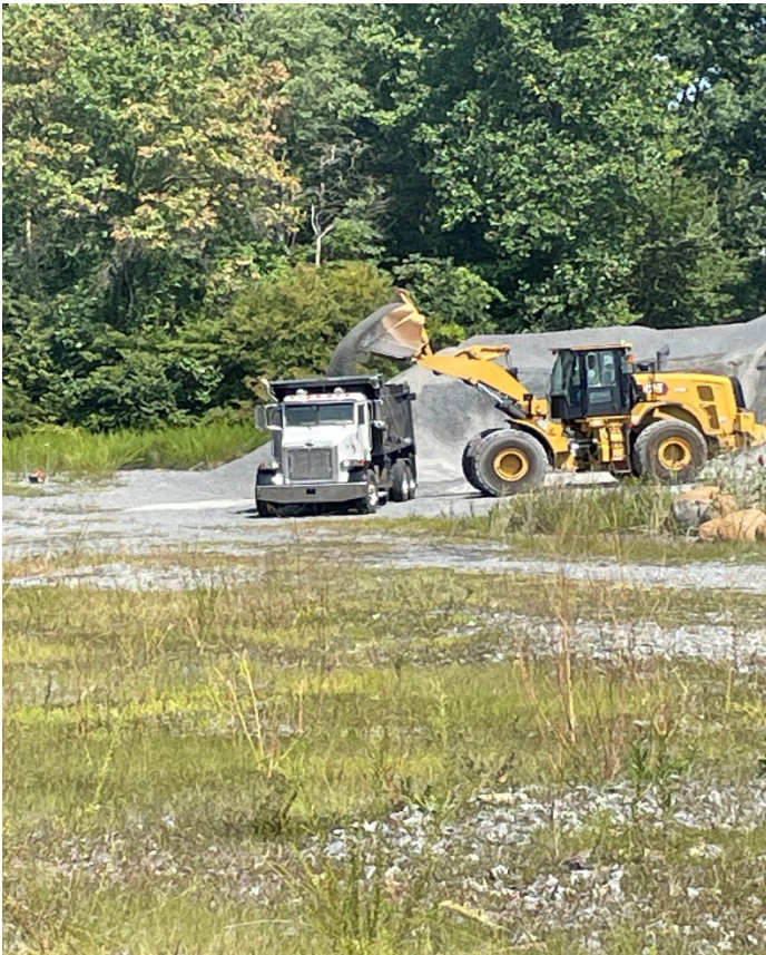
Rubber tire loader loading the truck with aggregate from stockpile- 8/22/23, 1136am
