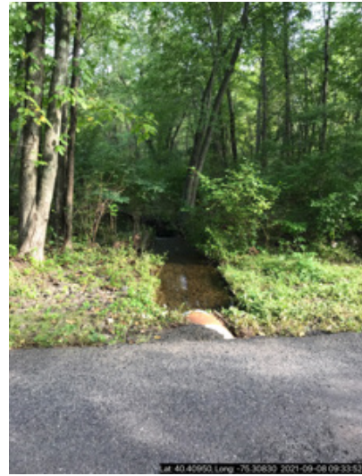
Outlet side of Rockhill Rd
