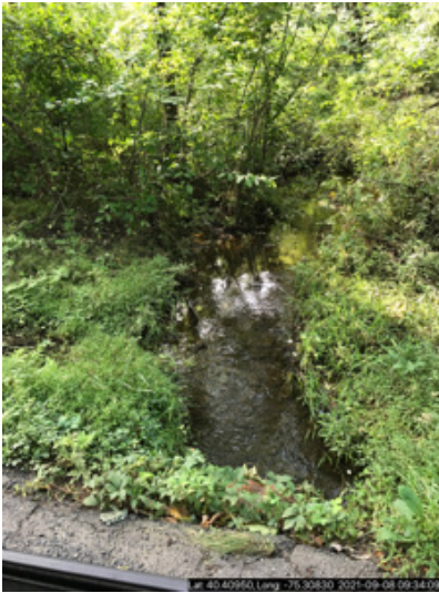
Inlet side of Rockhill Rd
